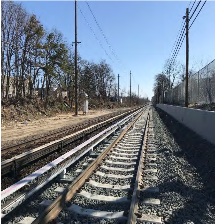
Force Account 3 rd Rail Installation just east of Rt. 111
