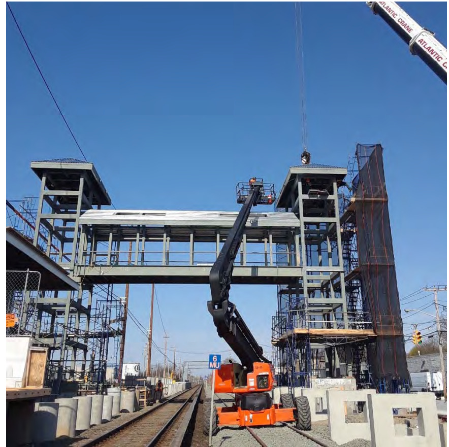
Installation of New Overpass at Wyandanch Station
