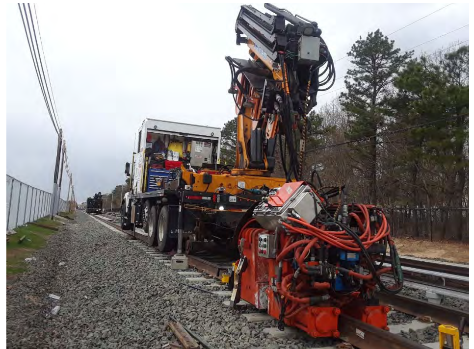
Rail De-Stressing and Welding
