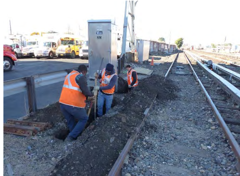
Conduit Install for New Electric Switch Heaters
