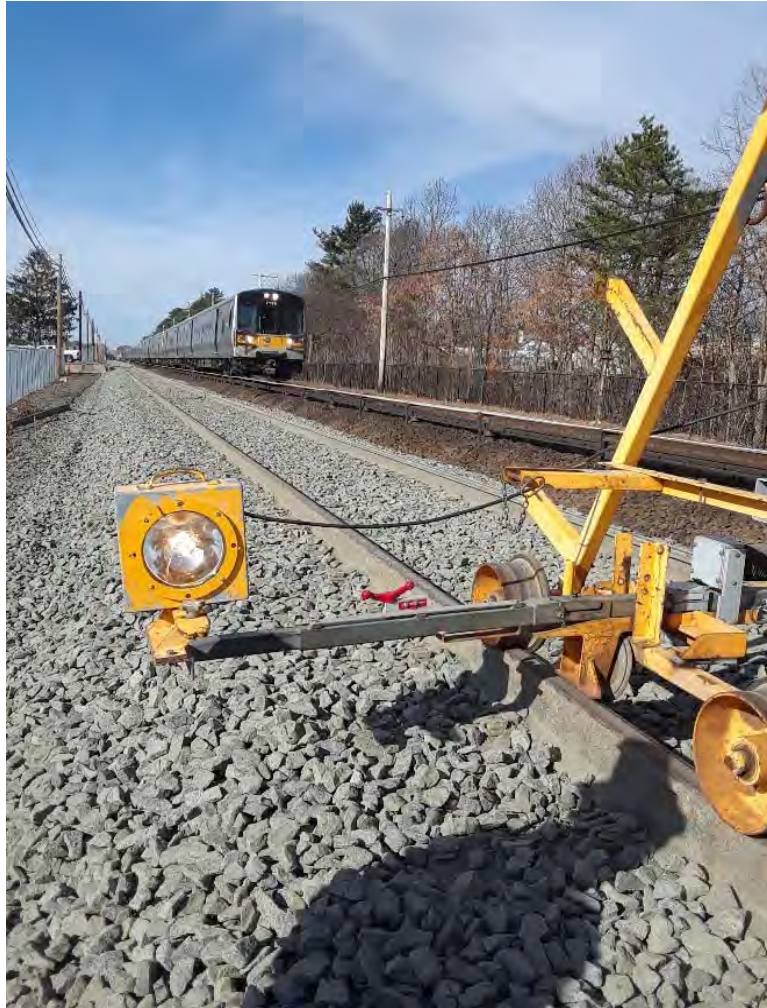
Surfacing of New Track West of Brentwood Station
