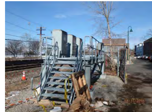
Sectionalizing Switches set on support platform at Irvington
