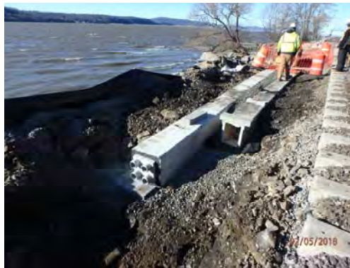
Precast conc. signal power duct bank/C&S troughs installed side by side.
