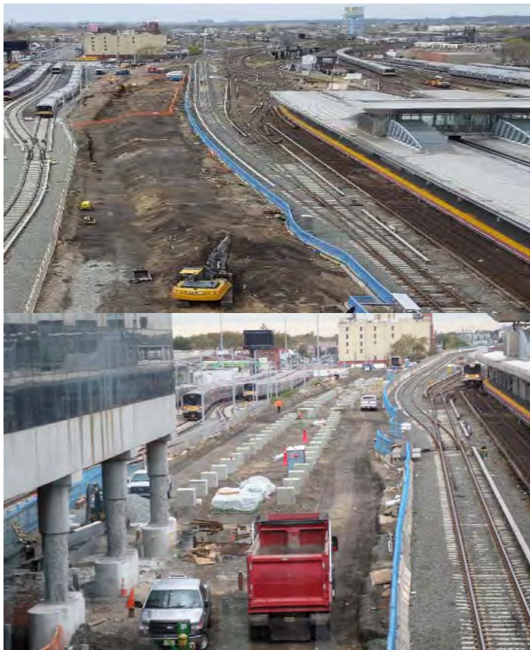
Platform Pile-caps Installed (Winter 2018)
