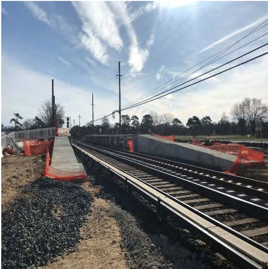
Track Installation and ADA Ramps at Pinelawn Station
