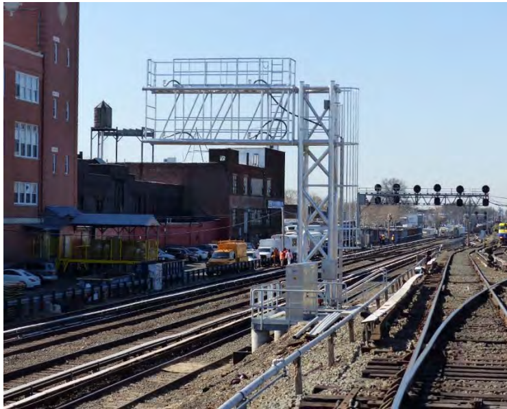
Dunton 3-Crossover New Signal Bridge
