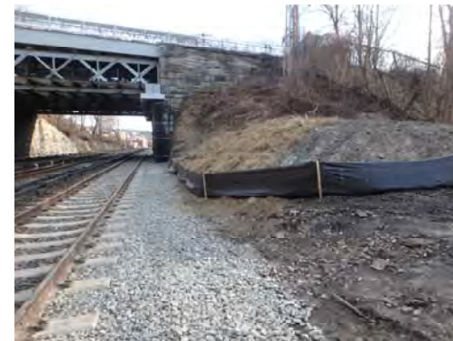
Right of Way restored (ballast and silt fence) North of Tarrytown
