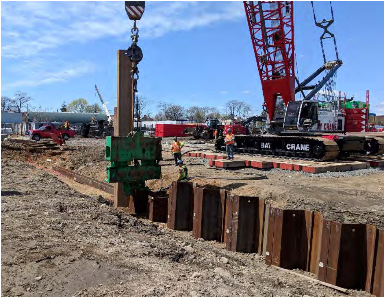
Sheeting Installation for Drop Pit Excavation
