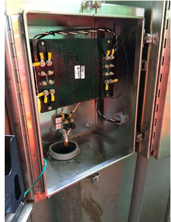
Antenna Pole/Radio Case/Communication Interface Case Installed at Tarrytown CP25
