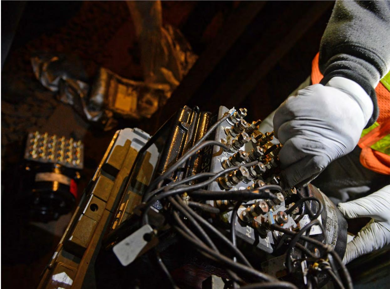
Maintenance on wayside track circuit relay which controls signal operations.
