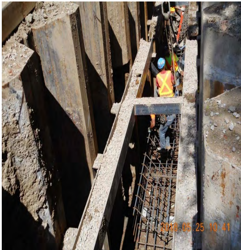
Rebar Installation for North Sewer Cradle between 1 st Ave & Ave A
