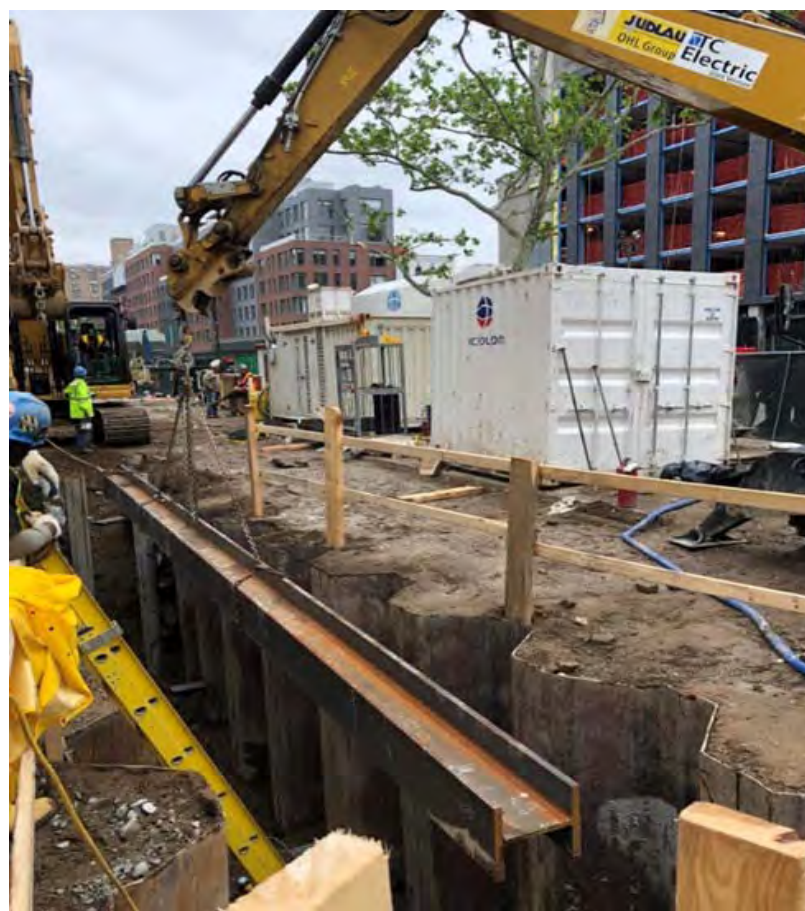
Installation of Steel Supports for North Sewer at Ave A & 14 th Street
