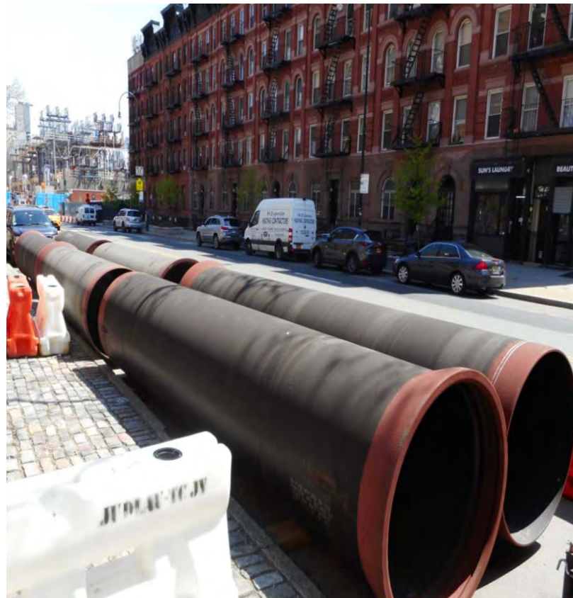
Delivery of 42" Ductile Iron Pipe for North Sewer at 14 th Street
