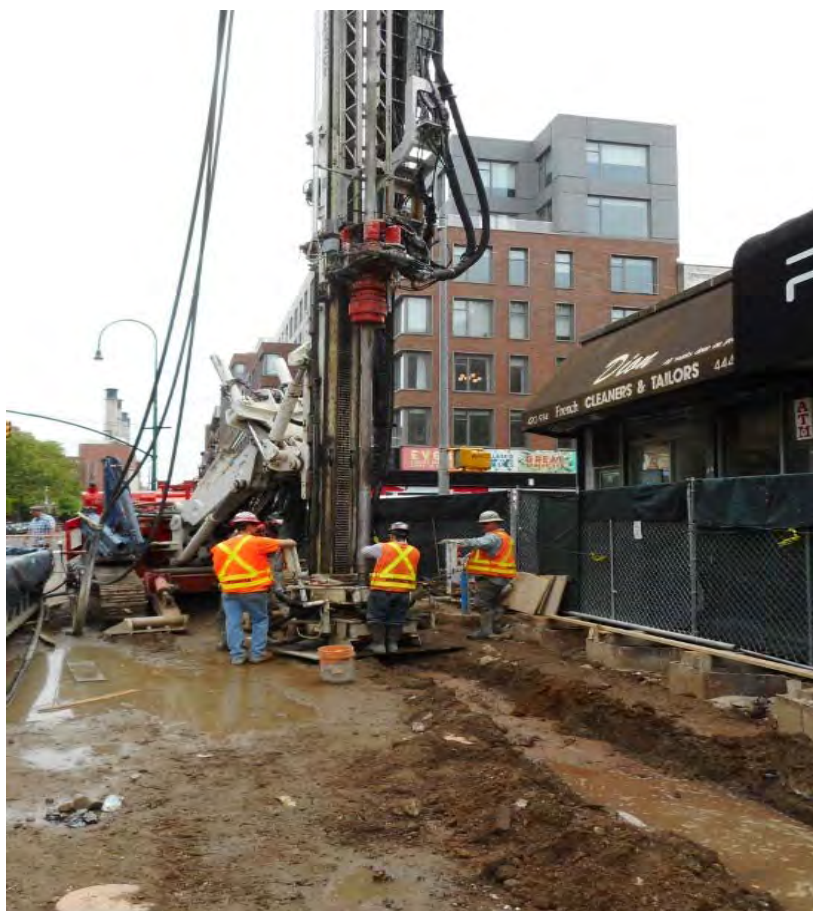
Jet Grout Installation for South Entrance at Ave A - 1 st Ave Station
