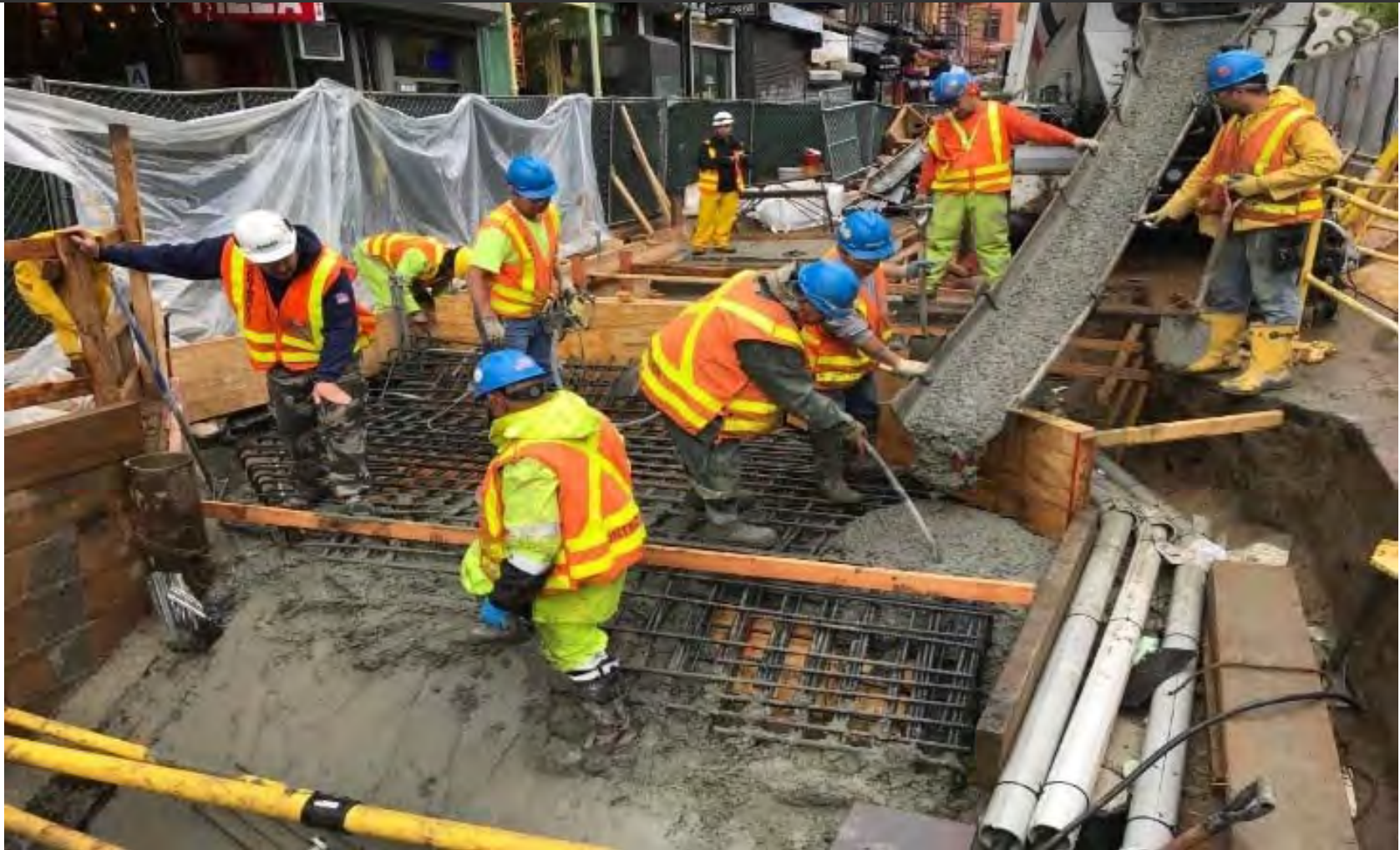
Concrete being placed for the roof of the New Bedford South Stair
