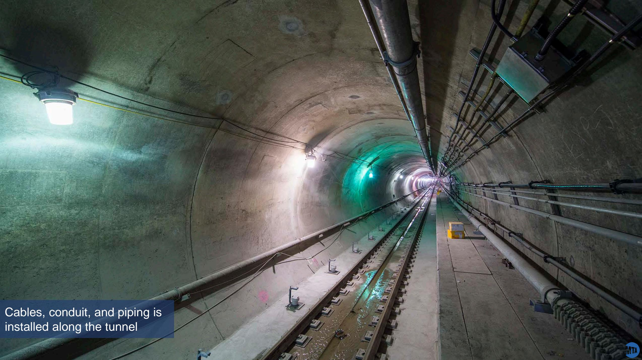
Cables, conduit, and piping is installed along the tunnel
