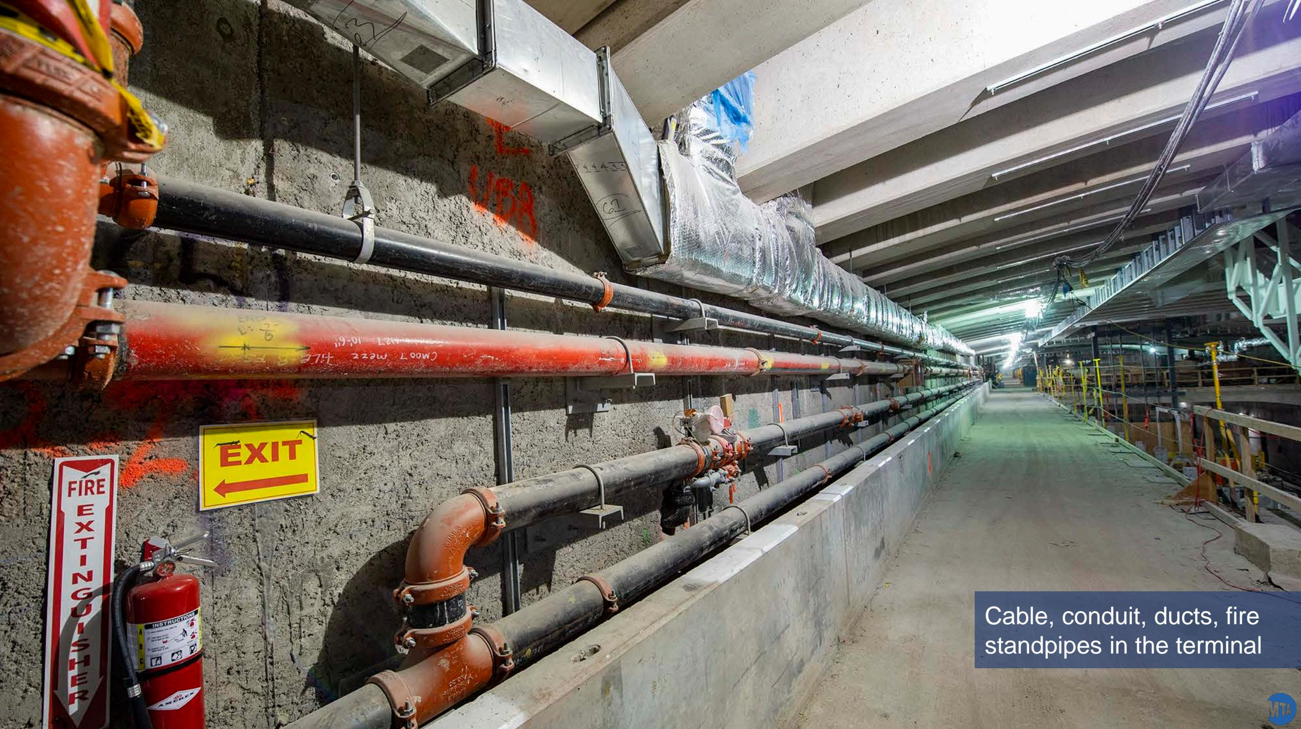
Cable, conduit, ducts, fire standpipes in the terminal
