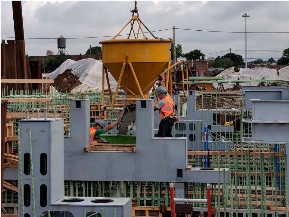
Concrete Placement of Drop Pit Foundation Walls
