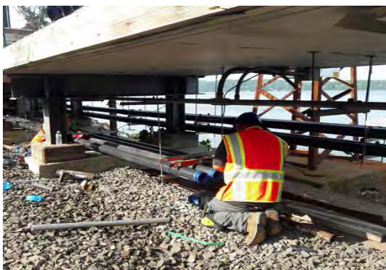
Conduits installation at Ardsley station underneath the platform
