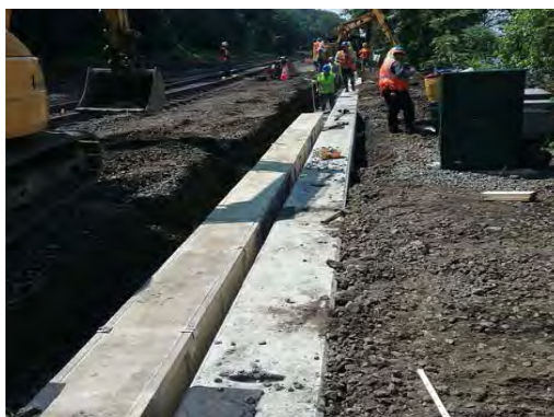
Side by side trough and duct bank
