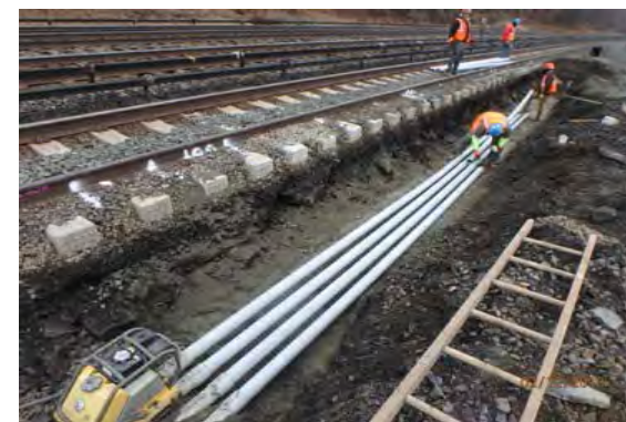
4" PVC conduit installation for Signal and Power
