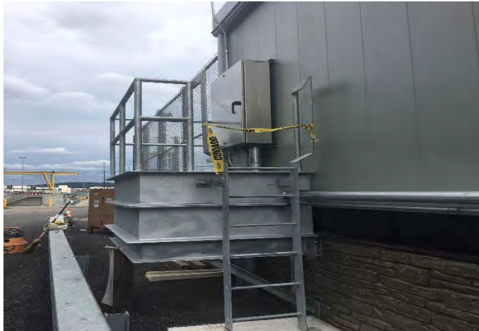
Installation of ladder at the platform at Croton-Harmon substation
