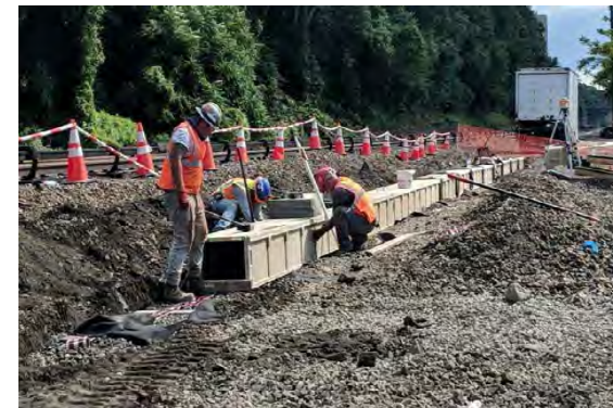
Trough installation at North of Greystone
