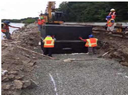
Installation of signal power manhole at Hasting
