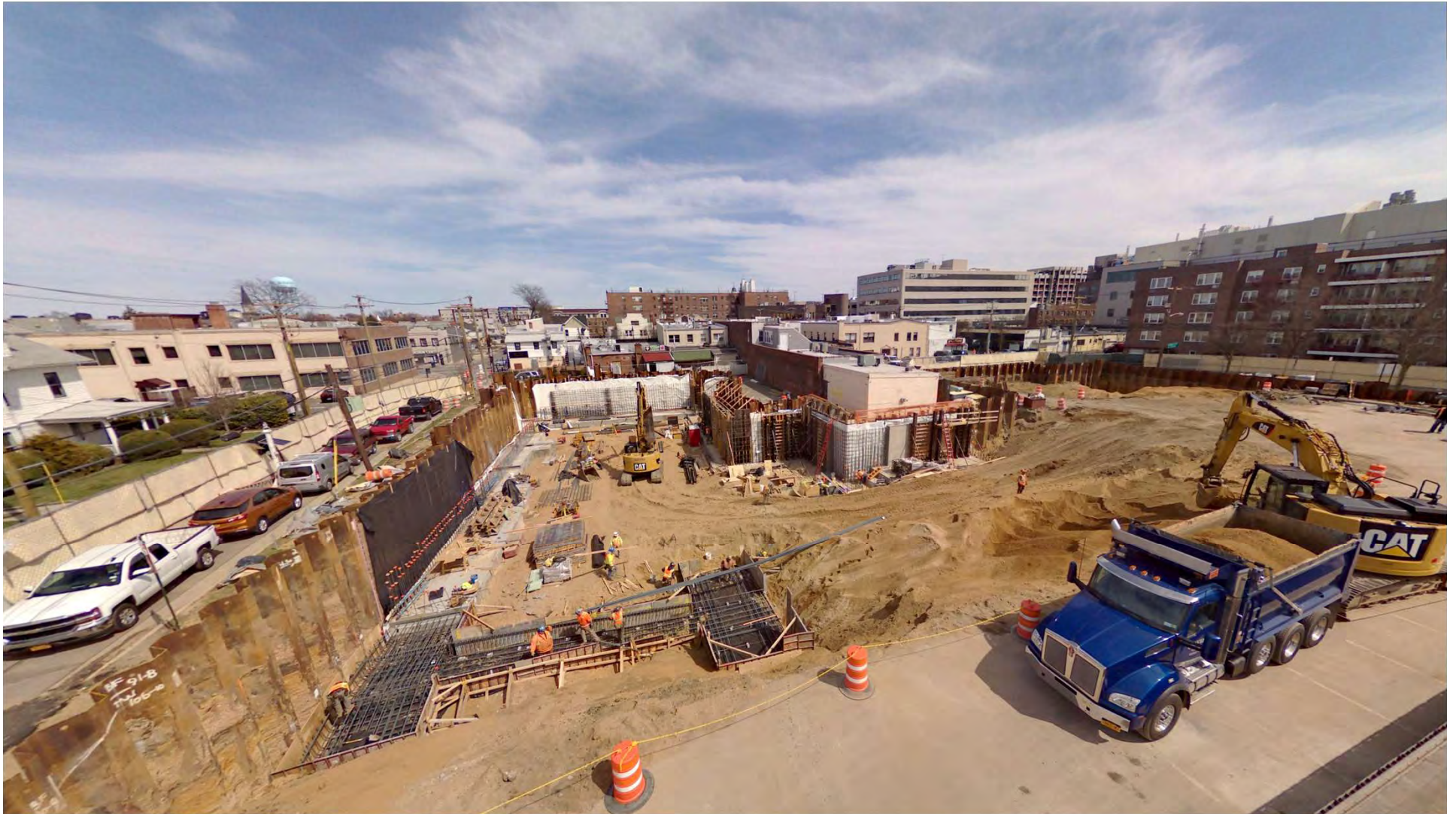
Excavating new foundations at Harrison Avenue Parking Structure in Mineola
