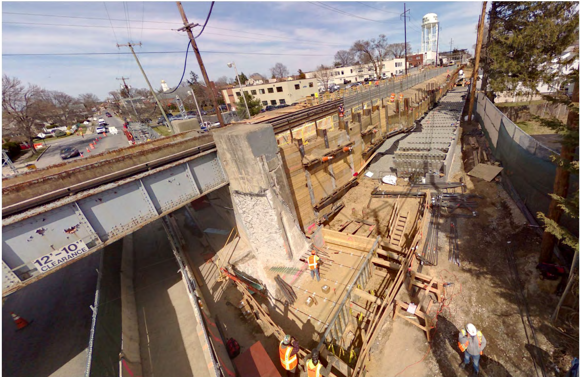
Excavation and SOE at Cherry Lane Bridge
