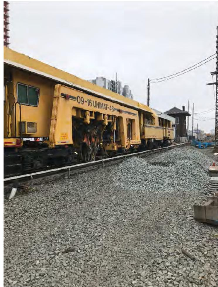
Realignment/Resurfacing of Track 10 by LIRR Forces
