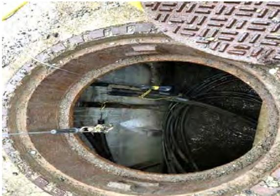
**Riverdale - Installation of 15kv jumper cables for Con Edison's metering work.**
