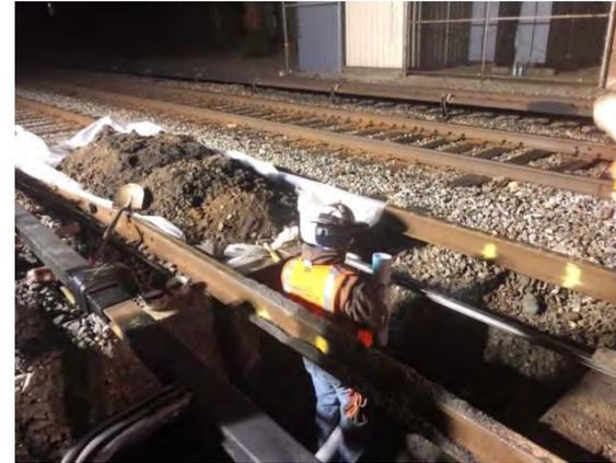
**Night Work:** Phase 1B – Hastings-on-Hudson North of CP19 Greystone - Crossing for track 2 Impedance bond conduits installation for traction power negative returns.
