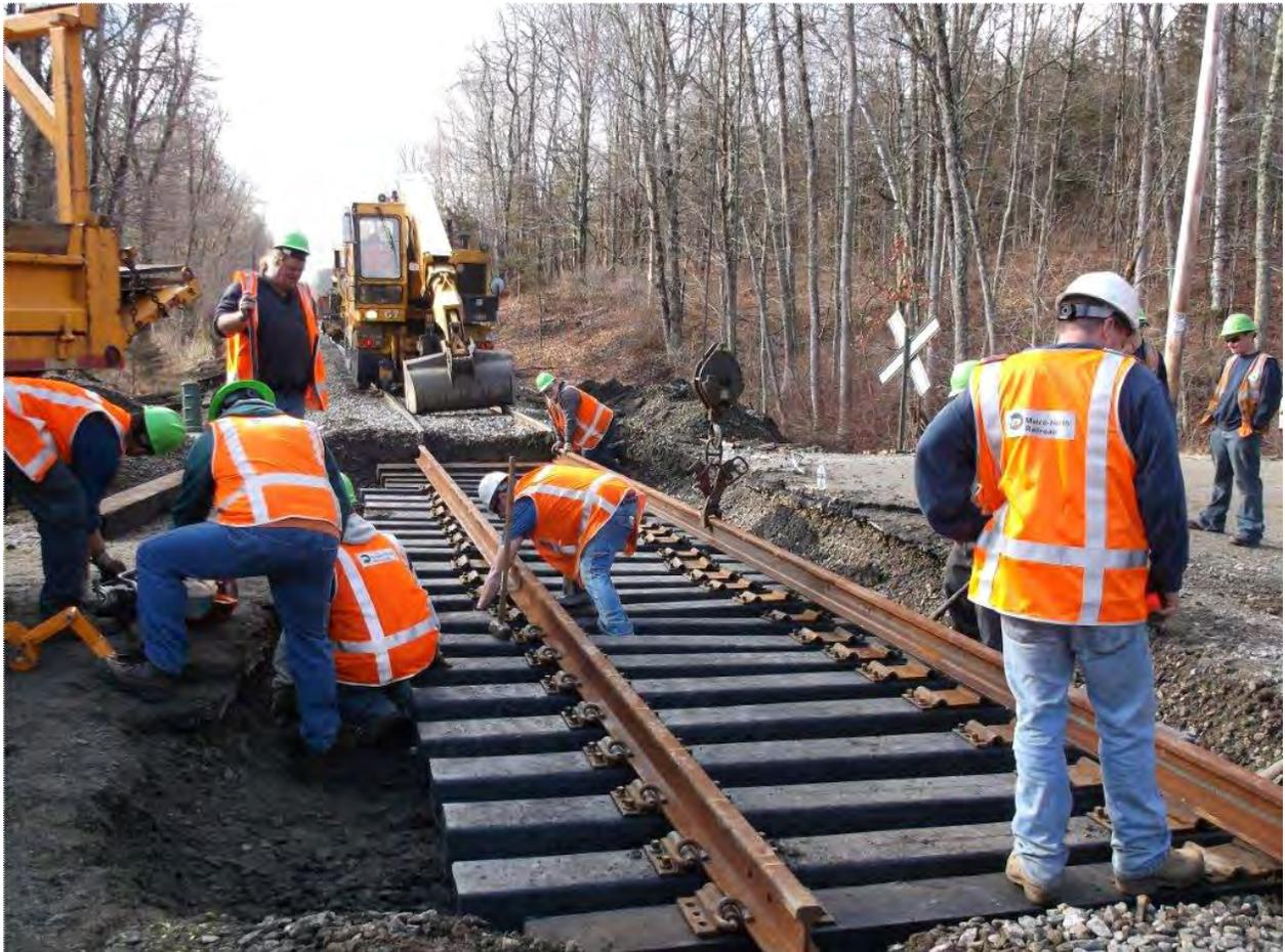
*Composite railroad ties have been used at Metro-North since 2014 as a replacement for old wooden and concrete railroad ties at crossings. Composite plastic ties last for approximately 50 years at crossings, which is significantly longer than traditional wood or concrete ties.*
