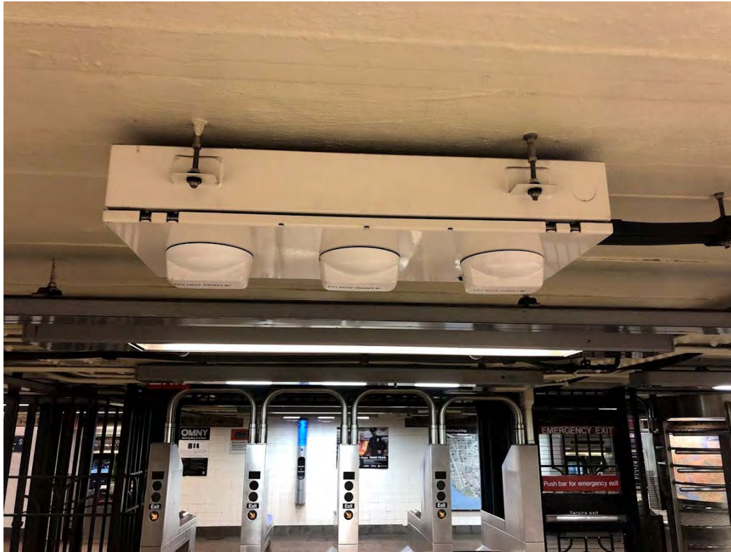
Cellular & Wi-Fi antenna mounted on mezzanine ceiling
