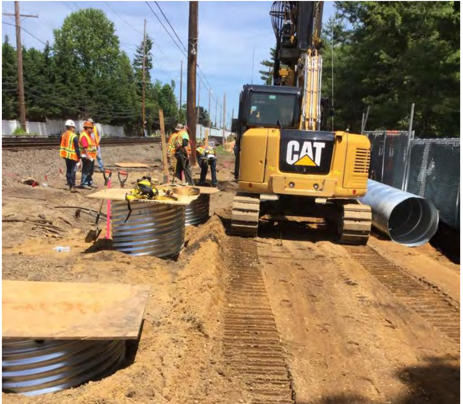
Caisson installation for sound walls around Nassau 1
