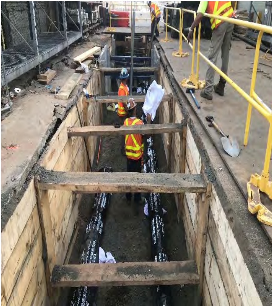
New Utility Tie-ins for Building "B"
