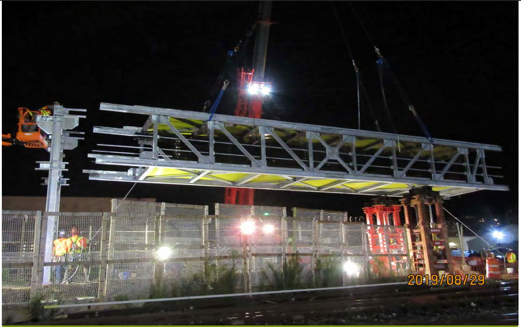
First Section of Cable Bridge Delivered & Installed
