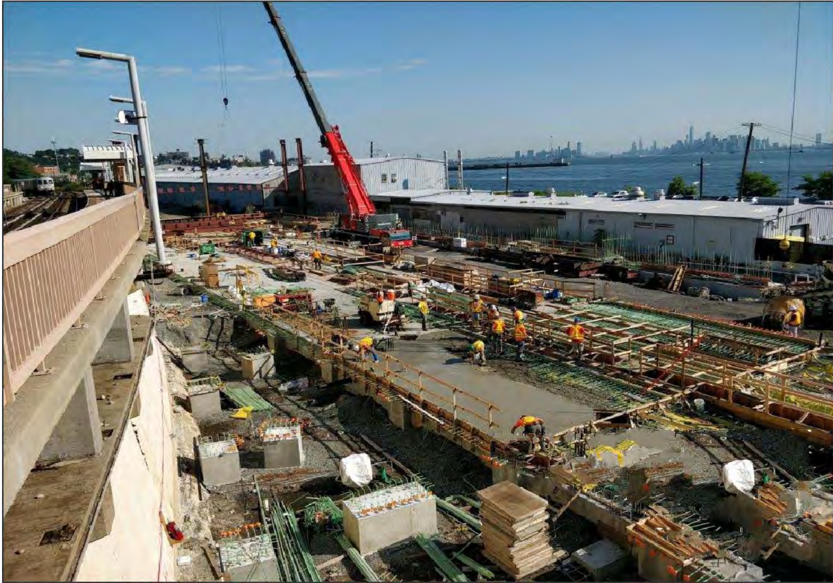
Concrete pours and start of steel erection
