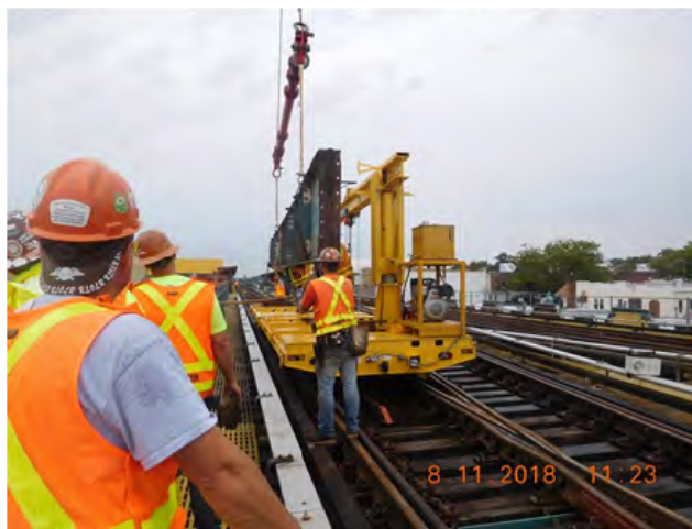
Removal of Existing Girders
