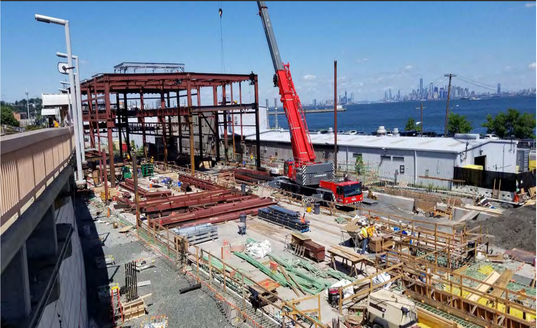
Steel erection and metal deck installation North to South
