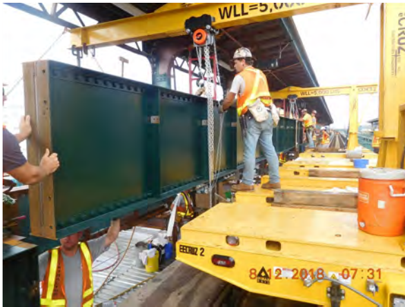
Installation of New Girders
