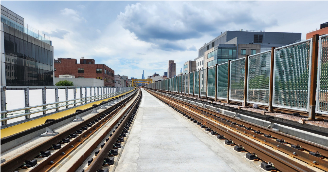
View at Track Level of the Completed Replacements of Tracks 3 & 1
