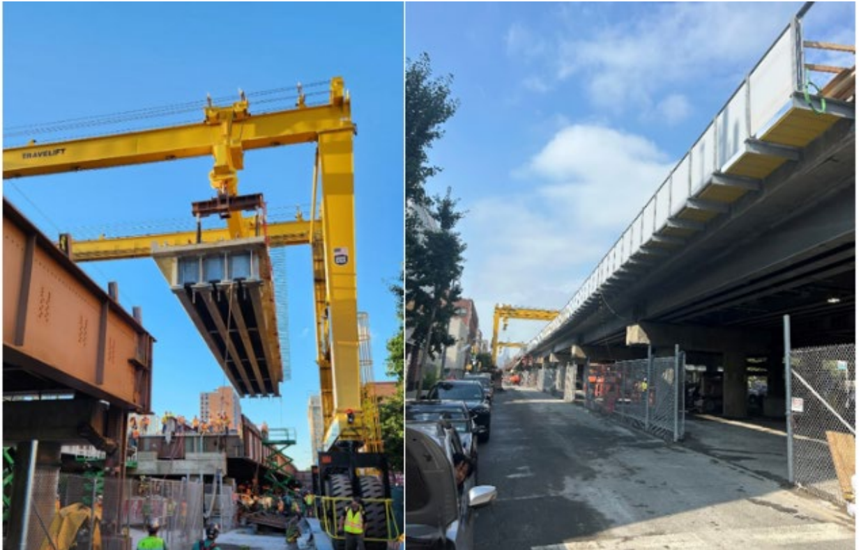
Gantry placing first prefabricated bridge unit (L.). New viaduct as seen from street level (R.)
