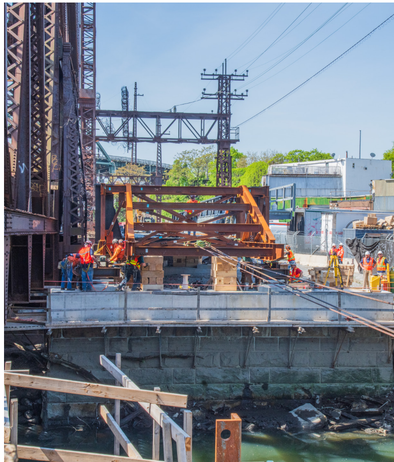
Crews using an air winch to launch Bronx River Bridge, May 2025
