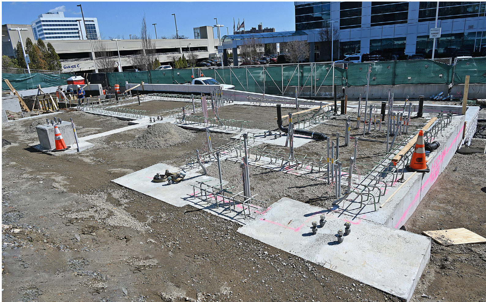
Foundation installation at Morris Park Station, March 2025
