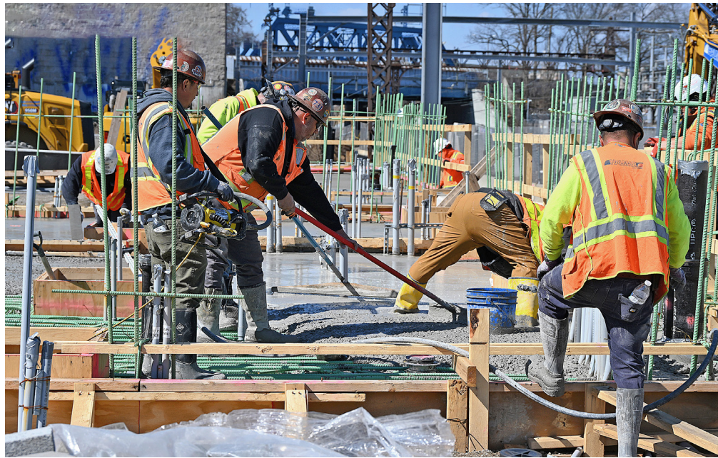
Concrete pour for entrance slabs at Van Nest, March 2025
