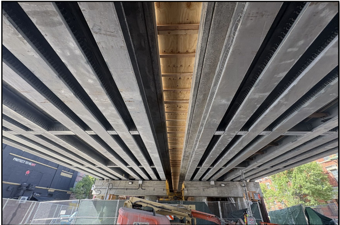
Underside of New Park Avenue Viaduct
