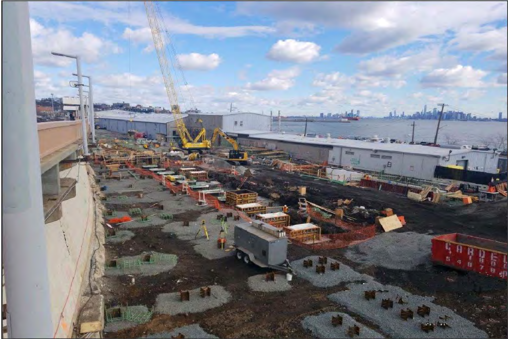
Pile Caps installed
