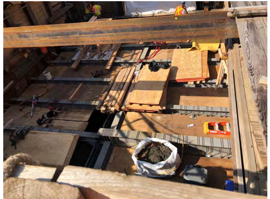
Shielded the South Excavation area
