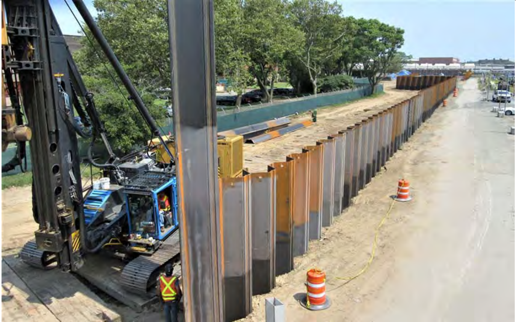
Perimeter Protection – Flood Wall along John Dewey High School in Stillwell Yard
