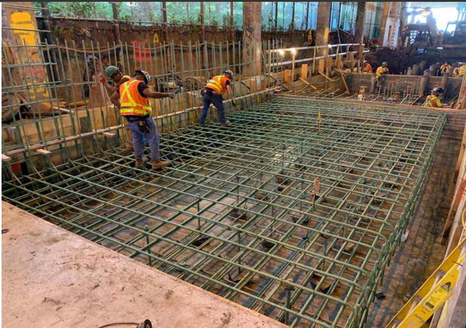
Construction of Footing for Flood Wall
