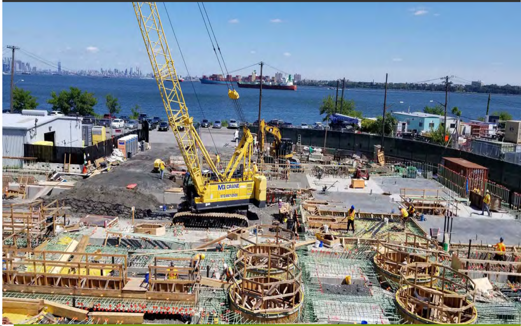
Front yard turntable form work
