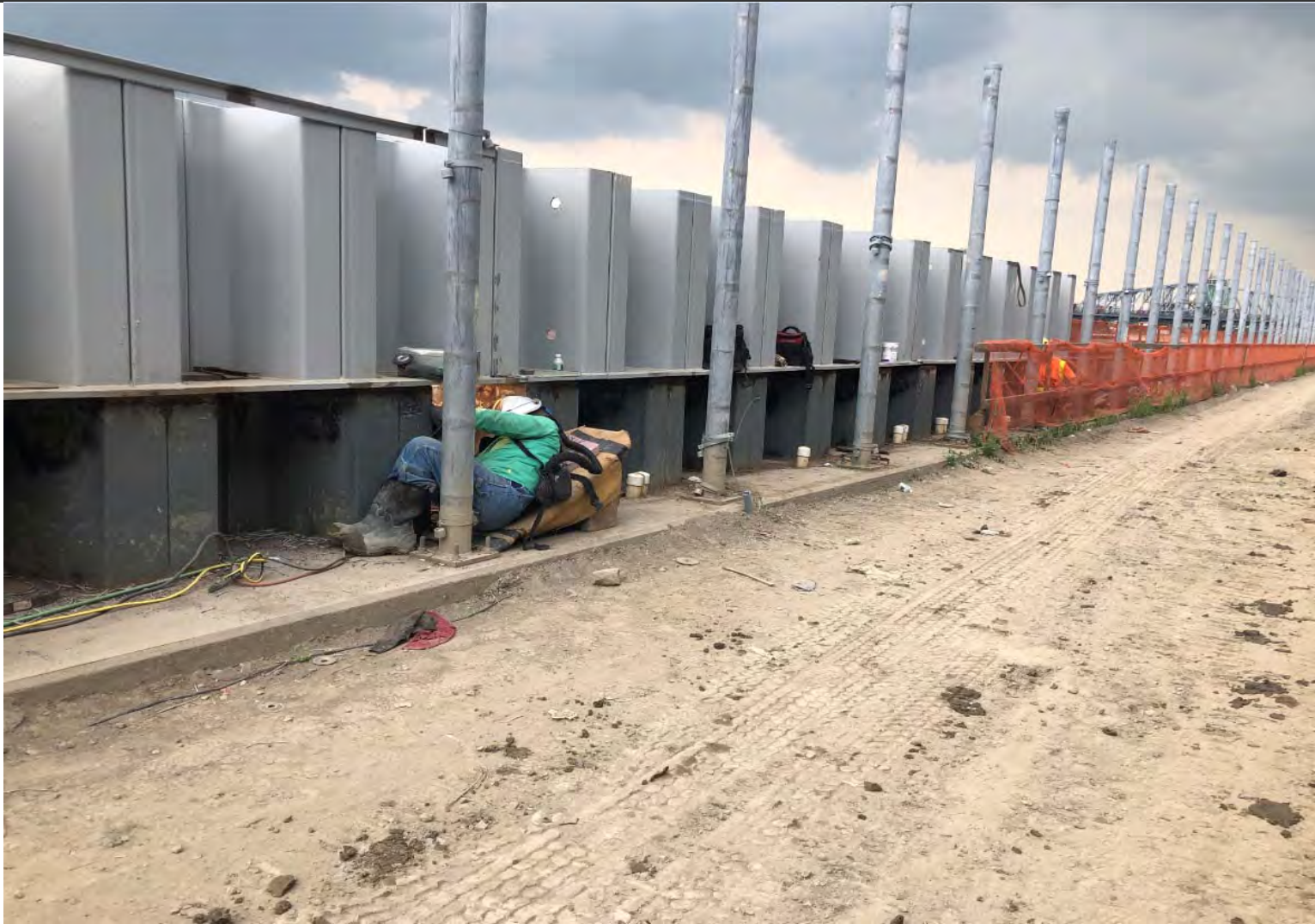
Installation of Sheet Pile Extension Adjacent to Harlem River
