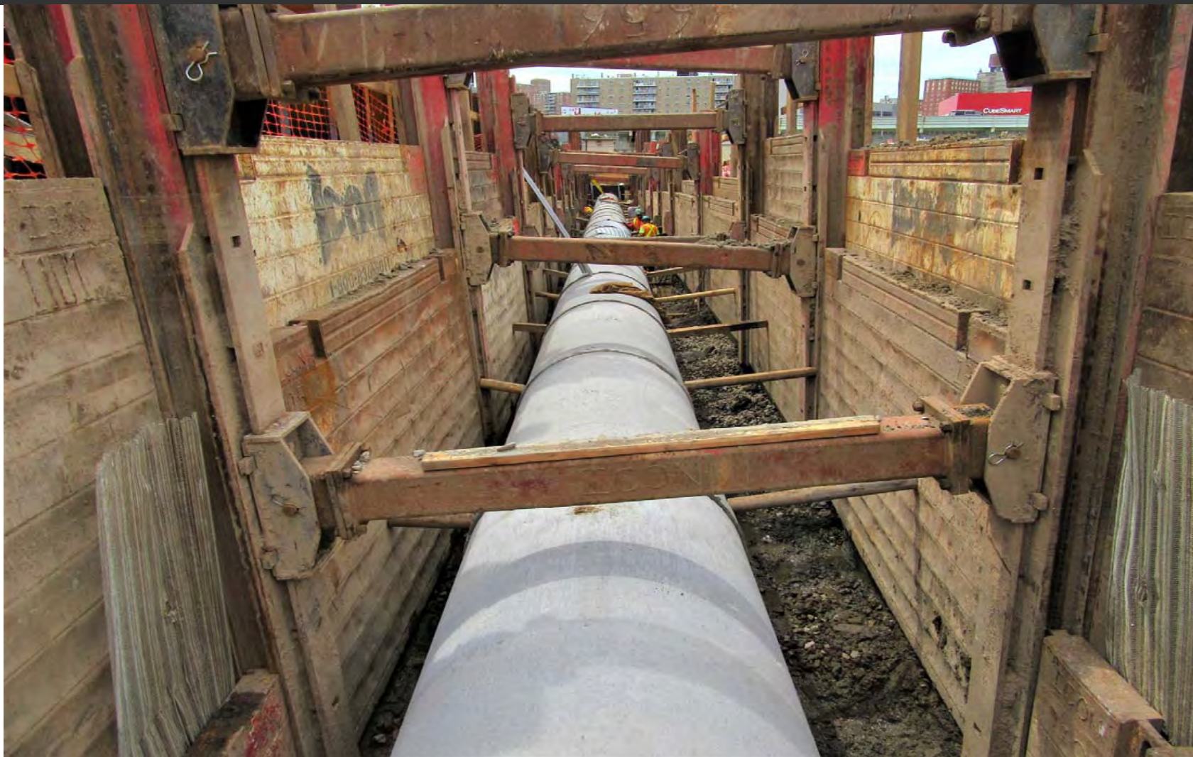
Installation of a new 42" Storm Sewer
