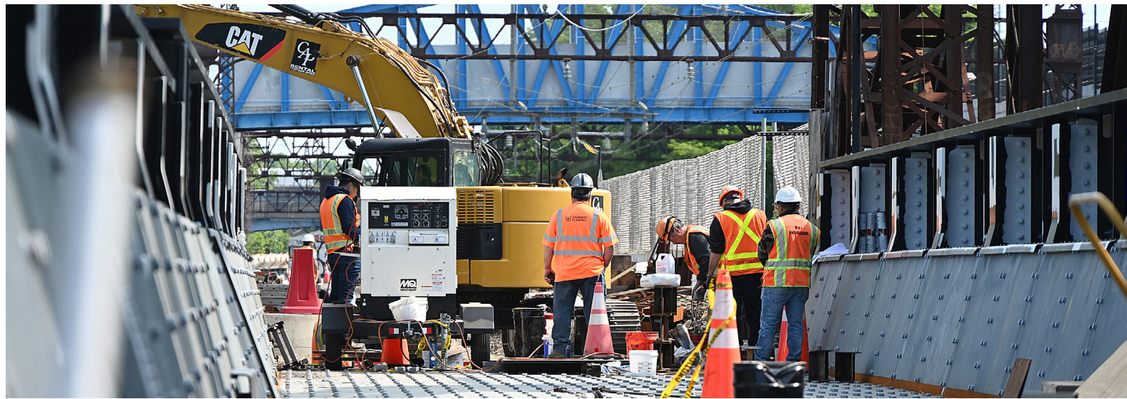
Backfilling approach slabs on Bronx River Bridge, June 2025
