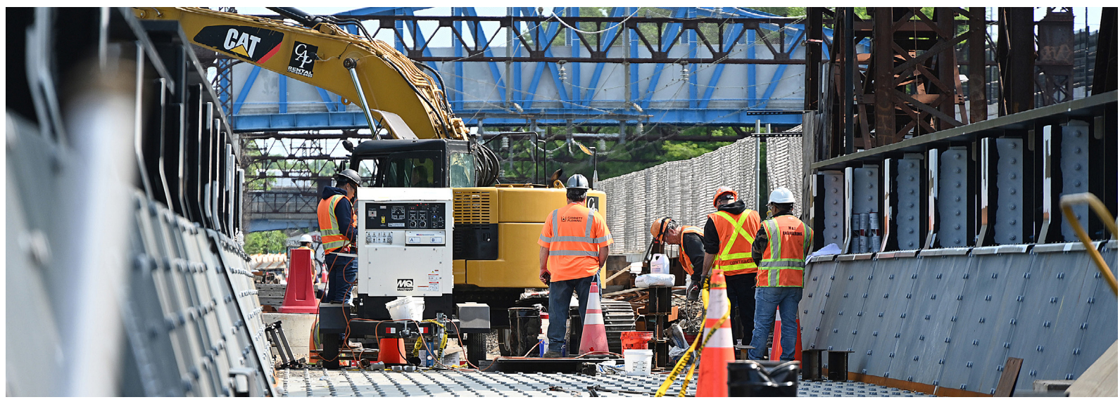
Backfilling approach slabs on Bronx River Bridge, June 2025
