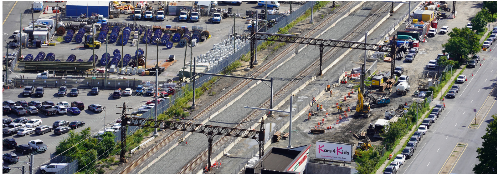
Overhead view of Parkchester/Van Nest Station progress, July 2025
