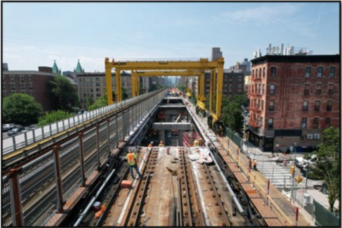
Removed Viaduct Deck Before New Prefabricated Bridge Units are Set
