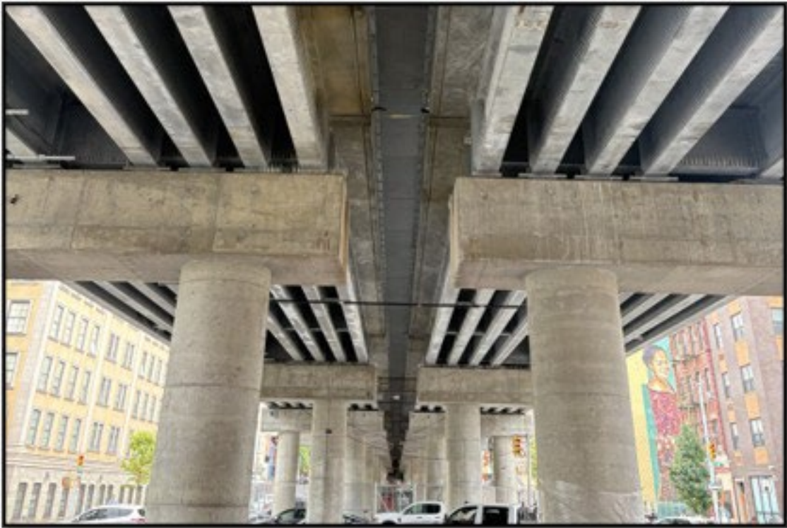
Underside of New Park Avenue Viaduct
