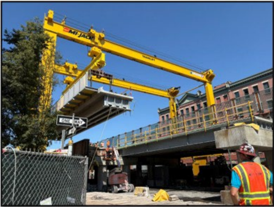
Setting of Outer Prefabricated Bridge Unit
