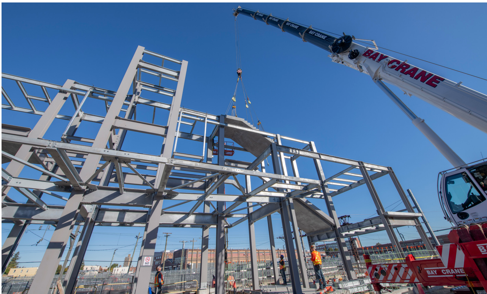
Steel framing at Parkchester Van-Nest station, October 2025
