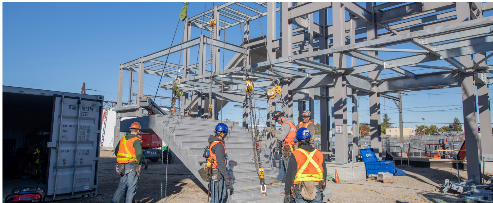
Concrete staircase installation at Parkchester Van-Nest station, October 2025
