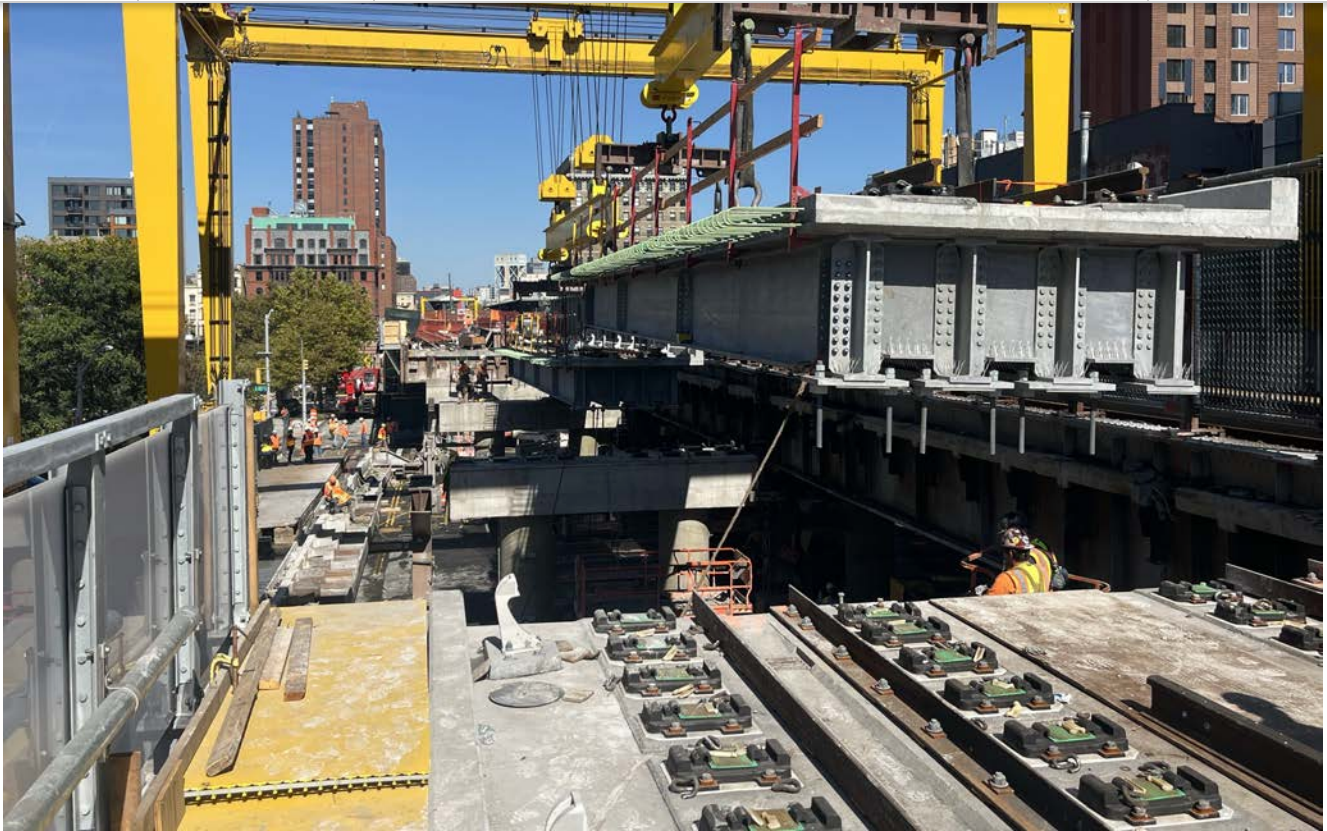
Gantry setting inner track during BRO 19
