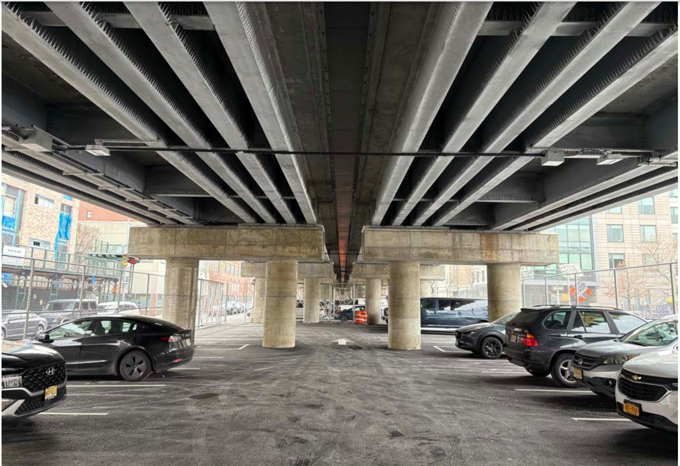
Underside of New Park Avenue Viaduct
