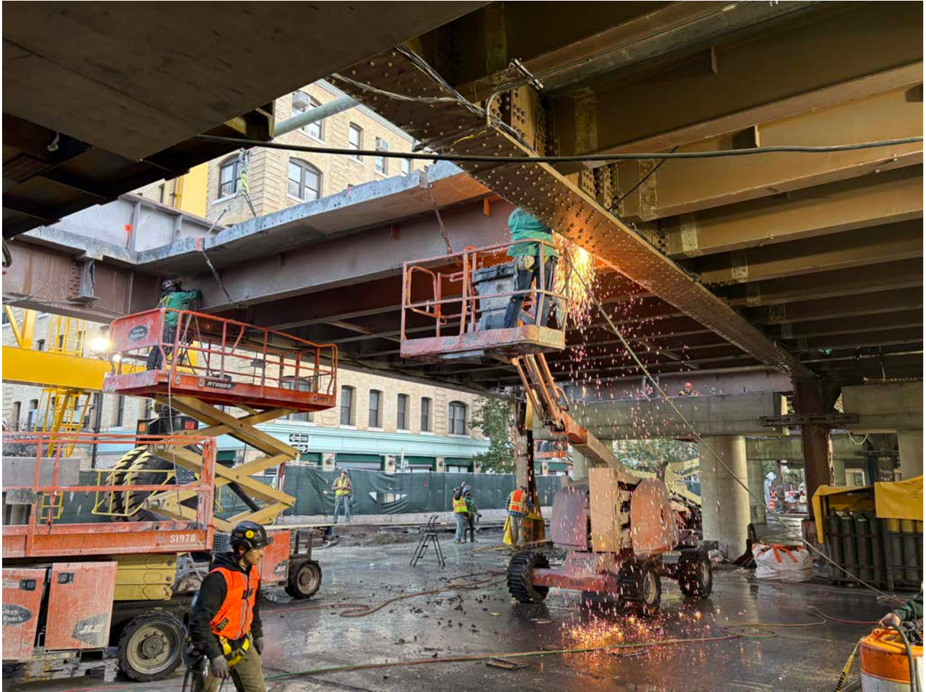
Plasma Cutting Steel for Removal of Viaduct Deck
