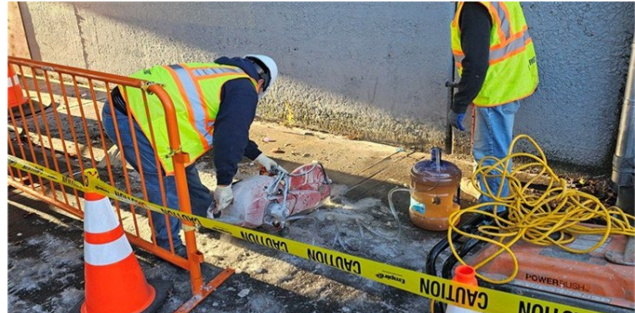
Test Pit Operations on Cypress Avenue
