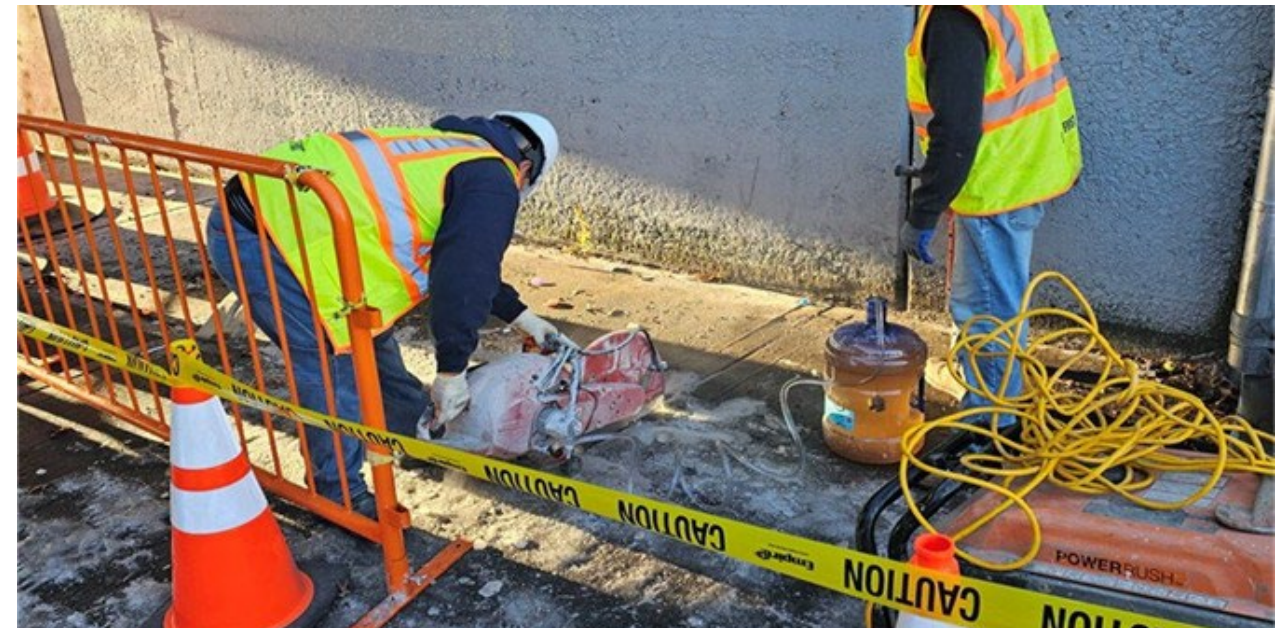
Test Pit Operations on Cypress Avenue
