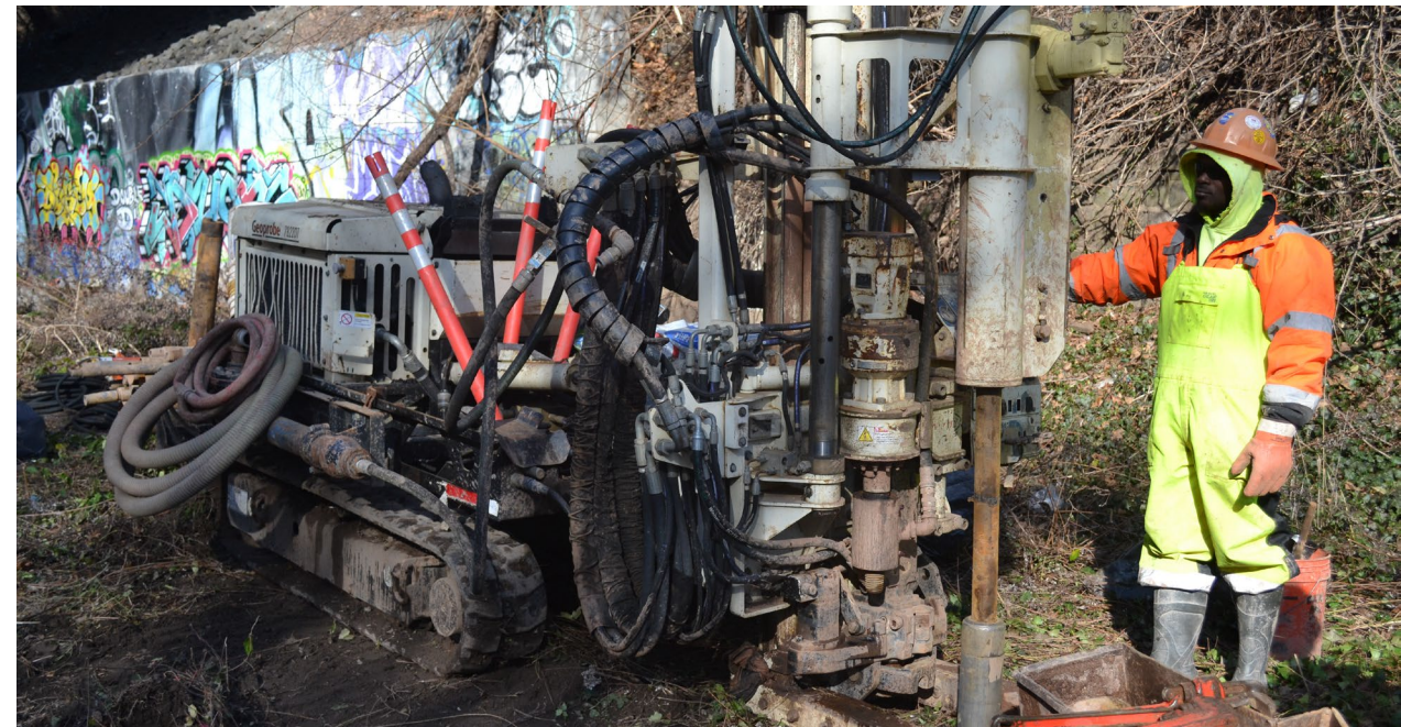
Soil Boring Operations within LIRR Bay Ridge Branch
