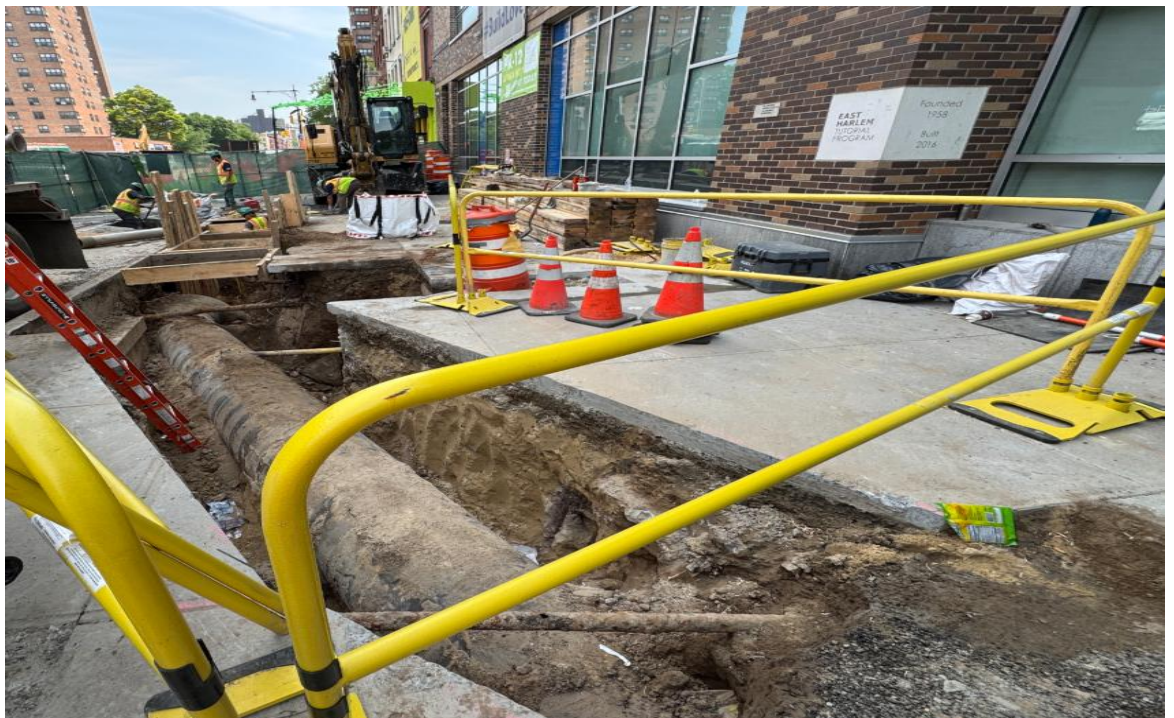
Excavation on 105 th Street and Second Avenue
