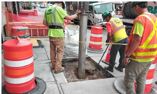
Utility Test Pits on 2nd Avenue Sidewalk
