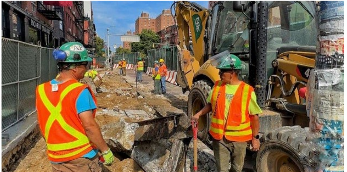
Sidewalk cutback: West side of Second Avenue
