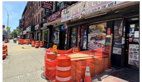
Utility Test Pits Between 109th and 110th
