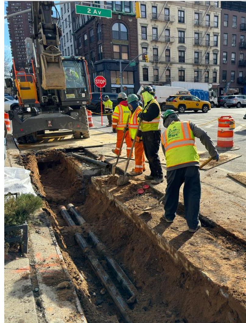
109th Street - 1st & 2nd Avenue- Electrical Duct
