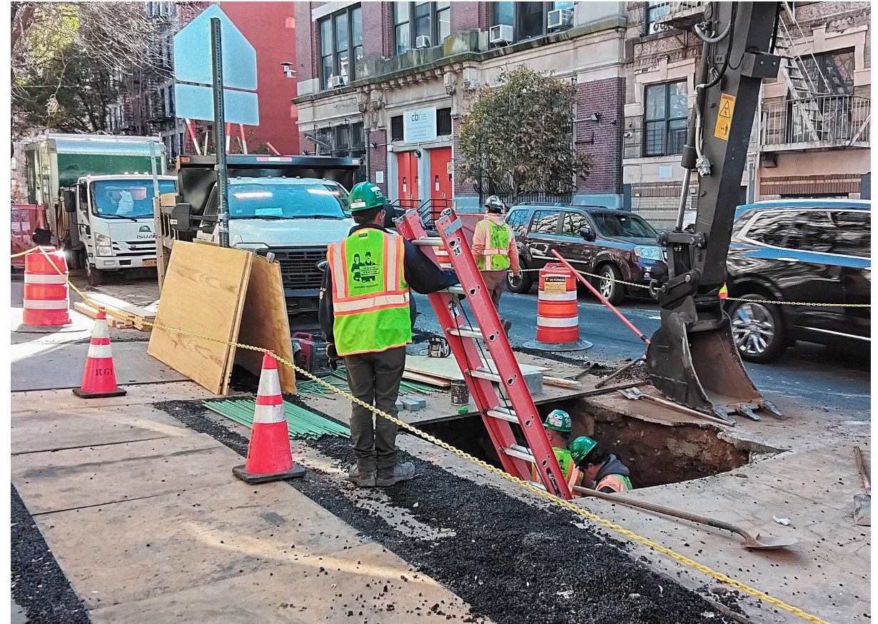
109th Street - 1st & 2nd Avenue- Electrical Duct
