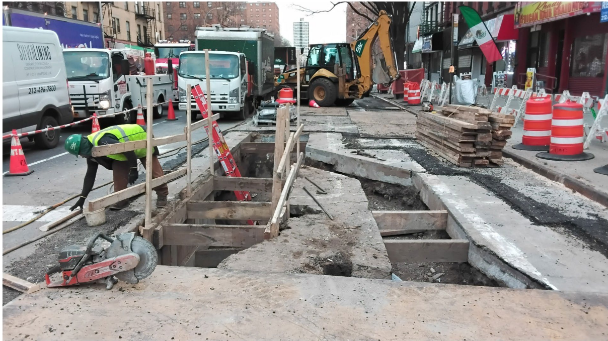
110 th Street, Second Avenue- Island Removal
