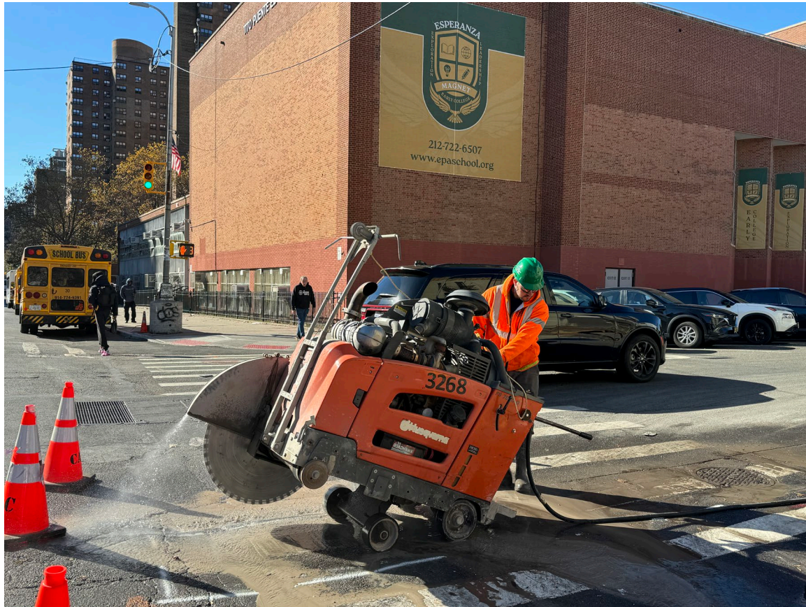
109th Street – 2nd & 3rd Avenue- Water main work
