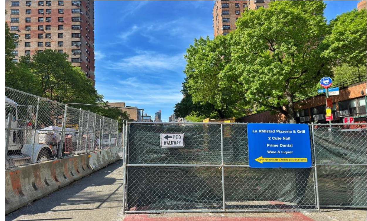
Corner MPT/Work Area 108 th St. looking south
