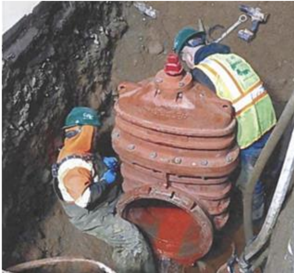
Water Main Valve Installation Throughout
