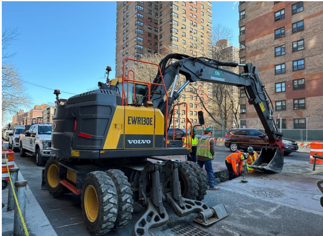
Fire Hydrant installation bet. 106 th and 107 th
