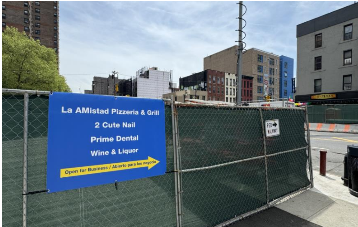
Corner MPT/Work Area 106 th St. looking east
