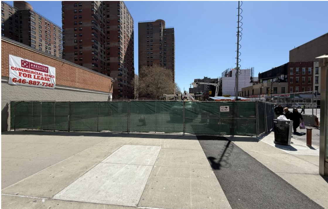
Corner MPT/Work Area 106 th St. looking east
