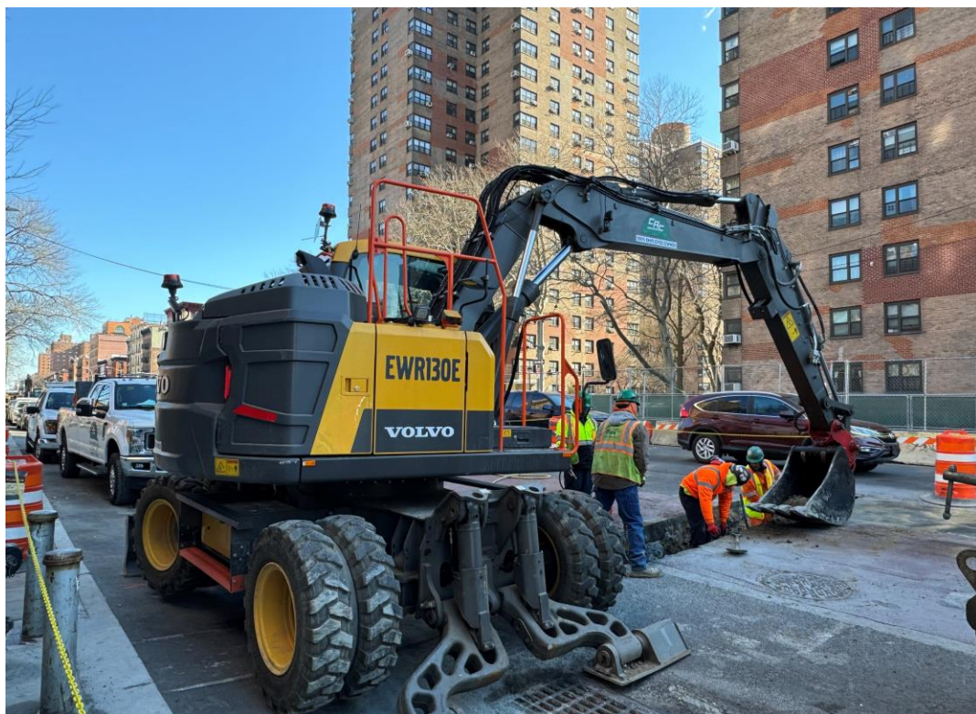
Fire Hydrant installation bet. 106 th and 107 th
