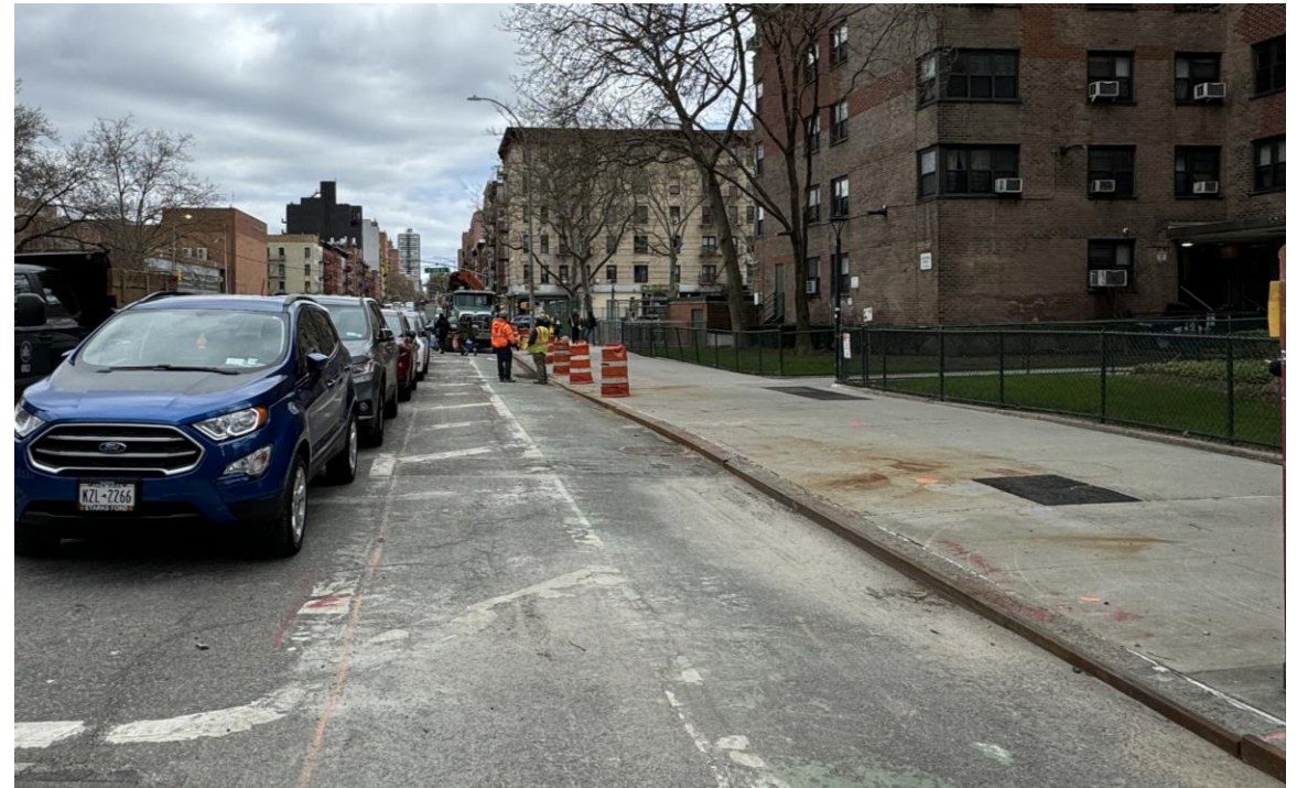
Work Area Removed
