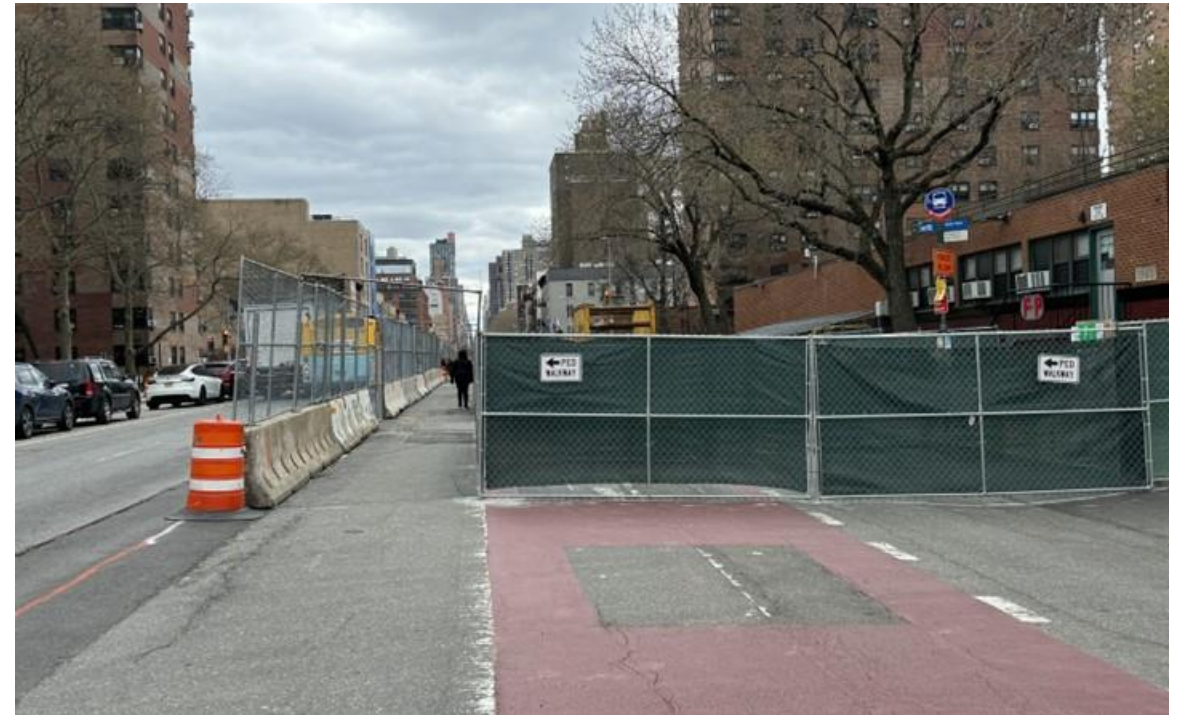
Corner MPT/Work Area 108 th St. looking south
