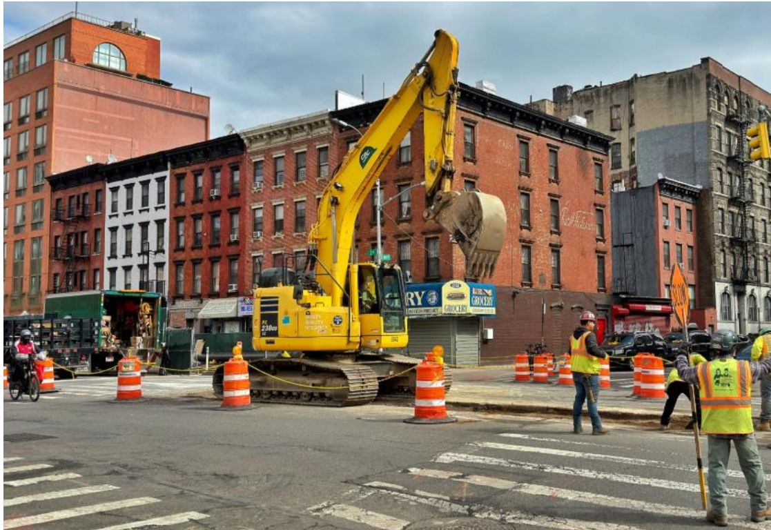
Water Main work at 109 th and 2 nd
