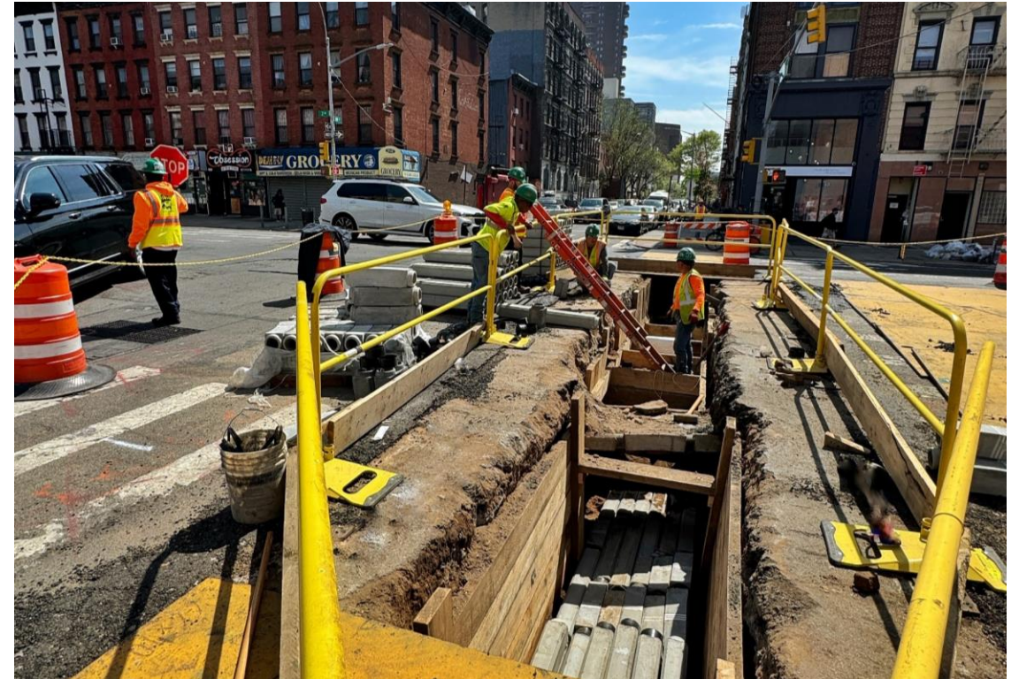
Electrical Conduit work 109 th and 2 nd
