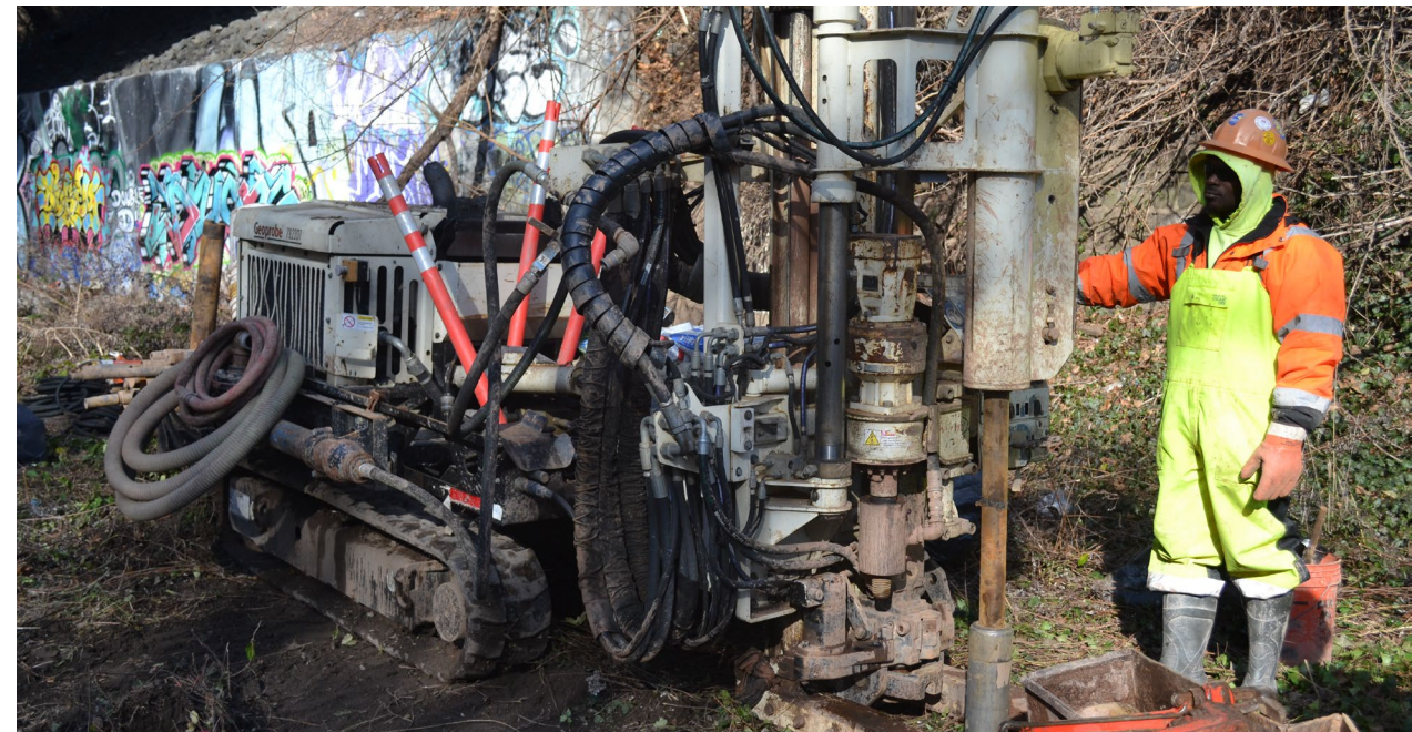
Soil Boring Operations within New York & Atlantic's Right of Way
