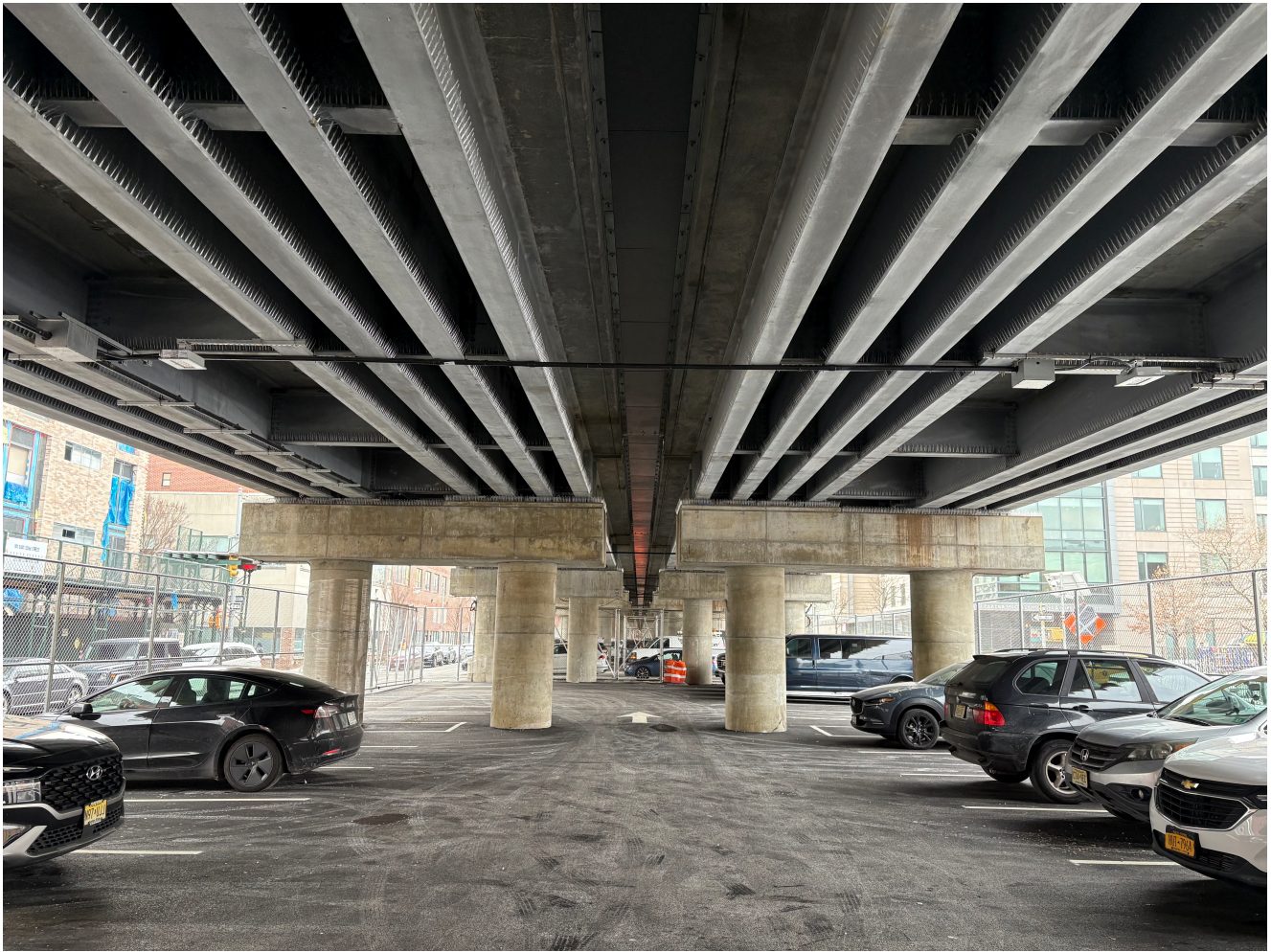
Underside of New Park Avenue Viaduct
