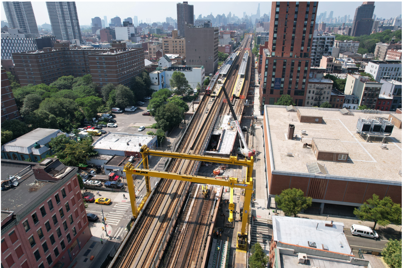
Aerial View of Phase 2 Replacement Circa 2025
