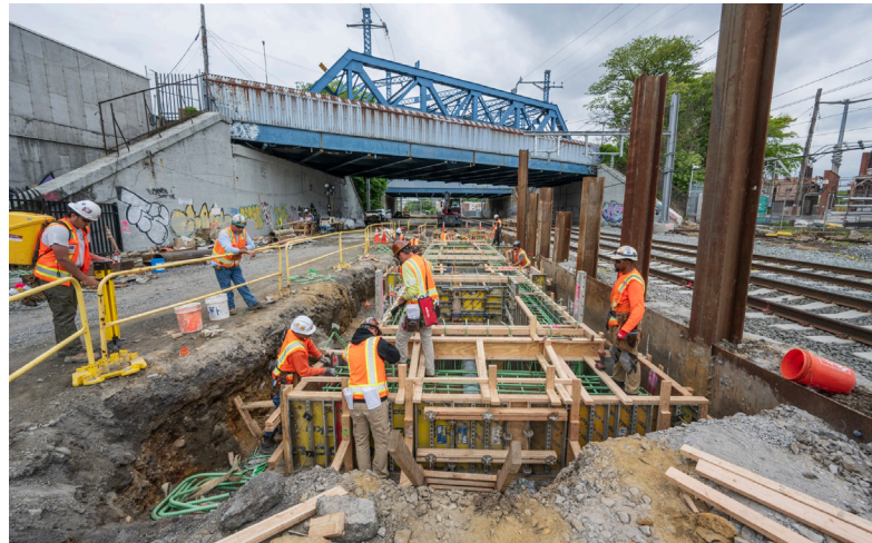
Installing formwork for concrete placement, May 2026
