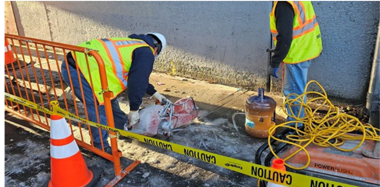
Test Pit Operations on Cypress Avenue
