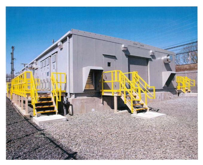
The picture above depicts the Long Island Rail Road's Meadowbrook Substation that was constructed utilizing the Design/Build method under Contract 6266. This month's agenda includes a procurement action for the award of a Design/Build contract for the replacement of Long Island Rail Road's Ocean Avenue Substation.
