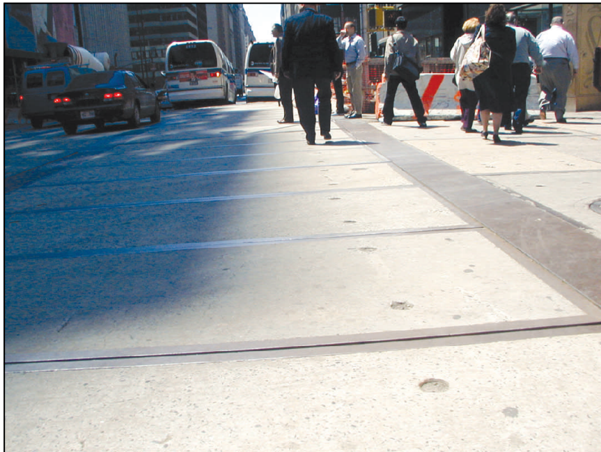
Example of cut-and-cover construction in place at Times Square
