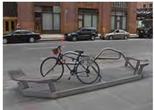
To keep pumps working well and to improve our ability to serve customers during intense rainstorms, we're now installing multi-purpose, raised grate "street furniture." This special furniture limits the flow of storm water into the subway and serves double-duty as public benches and bike racks.
