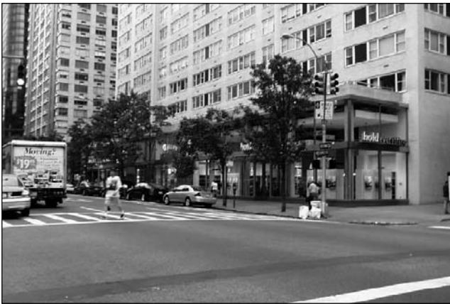
West side of Second Avenue, view south from 69th Street 3
