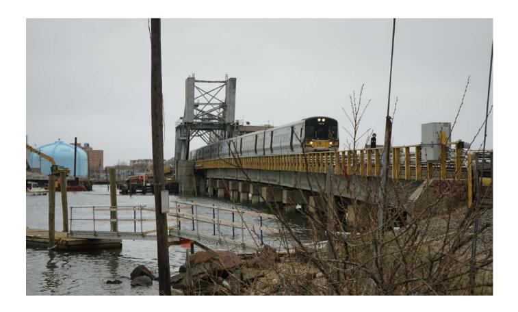
The picture above depicts a Long Island Rail Road passenger train traversing the Wreck Lead Bridge. The Wreck Lead Bridge carries passenger rail traffic on the Long Beach Branch over Reynolds Channel and connects LIRR service from Island Park to the City of Long Beach. This month's agenda includes a procurement action for the award of a construction contract to rehabilitate the moveable mechanical components of the bridge.
