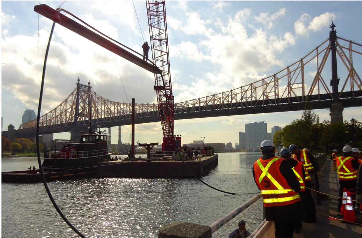
The 63<sup>rd</sup> Street Tunnel carries F trains between Queens and Manhattan and will serve future LIRR East Side Access trains. The unique construction of the tunnel requires a special cathodic protection system to prevent corrosion from the saltwater environment. Here, members of Subways' Maintenance of Way Power team use a barge and crane to install equipment at the bottom of the East River that was damaged during Superstorm Sandy.
