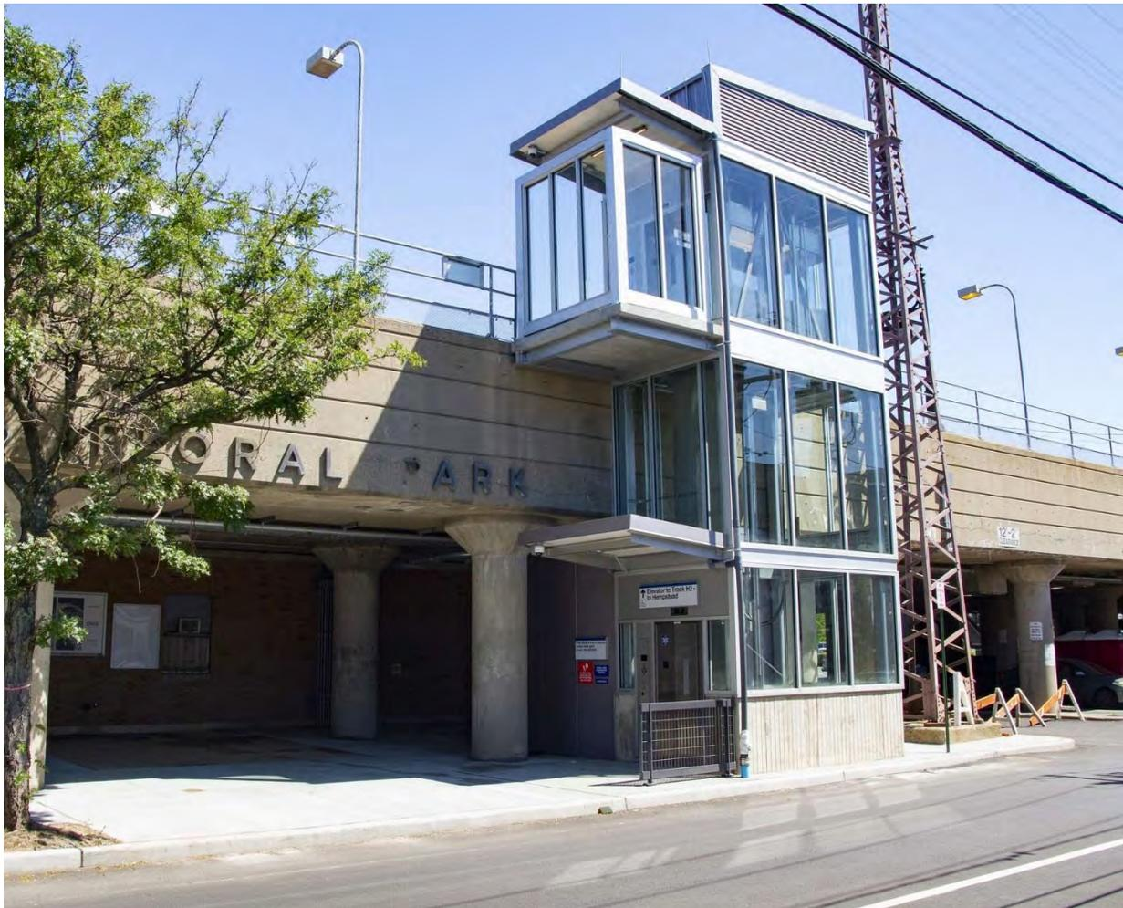
**ADA Accessibility:** Floral Park Station’s new elevators, which were installed to upgrade the station to be fully ADA accessible. This improvement is part of the Long Island Rail Road’s pledge to ensure full accessibility throughout the entire system.
