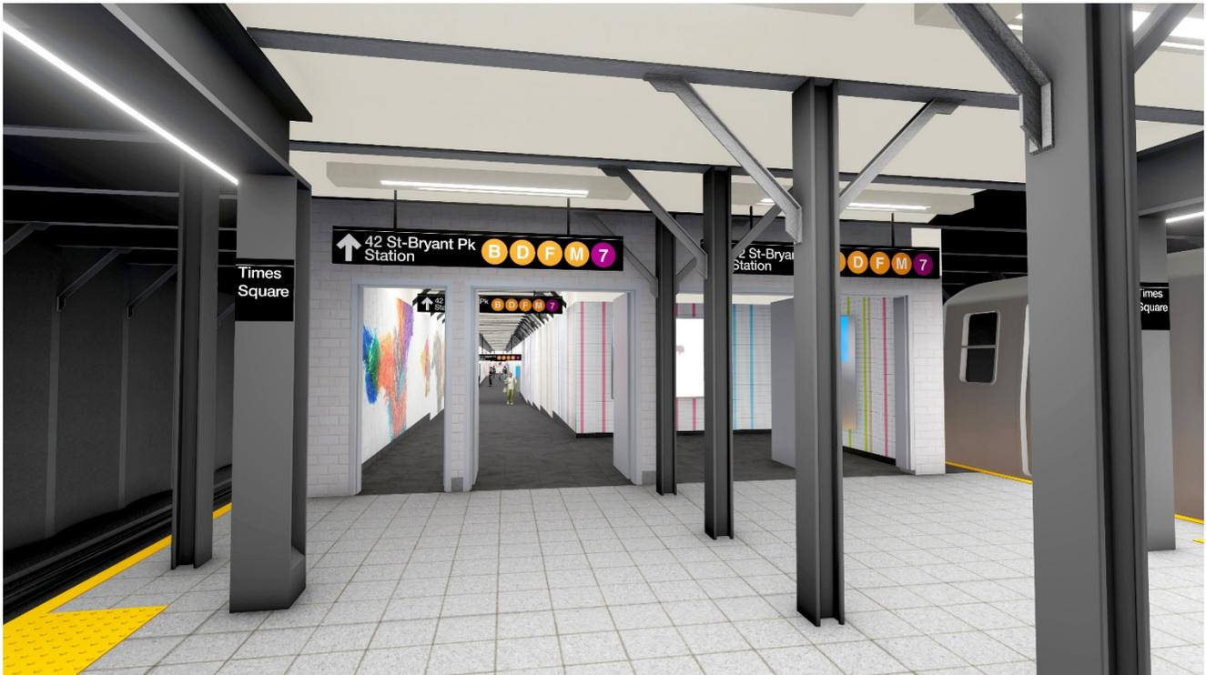
The above rendering depicts a new enclosed connector from the Times Square Shuttle's abandoned Track 3 Right of Way from the east end of the Times Square Shuttle platform to the Bryant Park Station. The procurement action required for this work is included in this month's procurement package.
