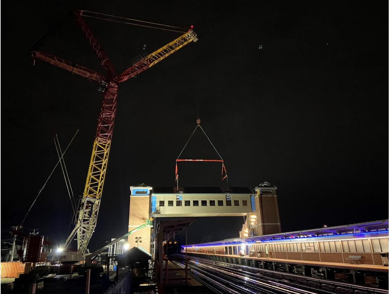
The picture above depicts the installation of the pedestrian overpass at the Elmont Station on the Main Line of the Long Island Rail Road. The work was done as part of Contract 6353 and took place over an outage during the weekend of March 18<sup>th</sup> – 20<sup>th</sup>.
